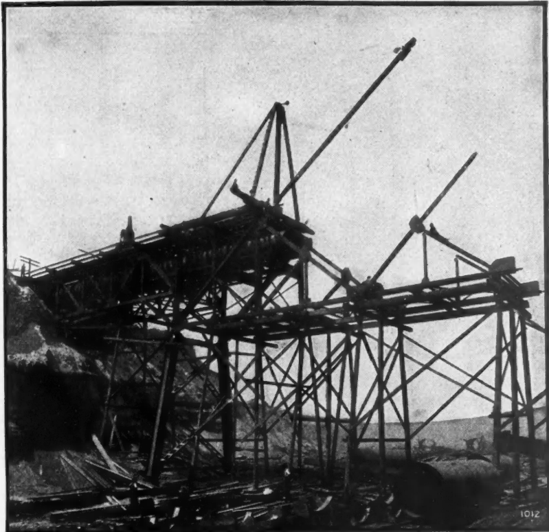
Erection of Highway Bridge Carrying Flume, Hibbing, Minn.
