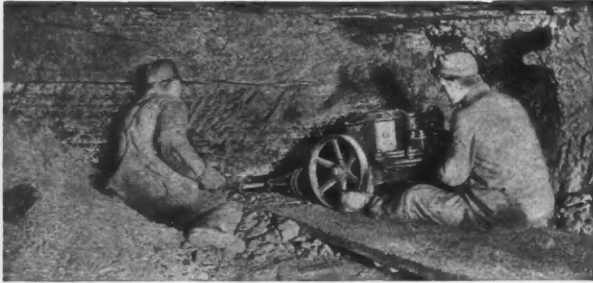
170 of these Electric Punchers in daily use at the mines where above photograph was taken.
