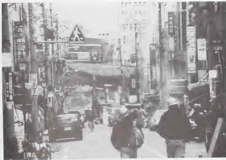
Figure 6.2.26 Collapsed train overpasses such as this one divided Kobe north and south.
