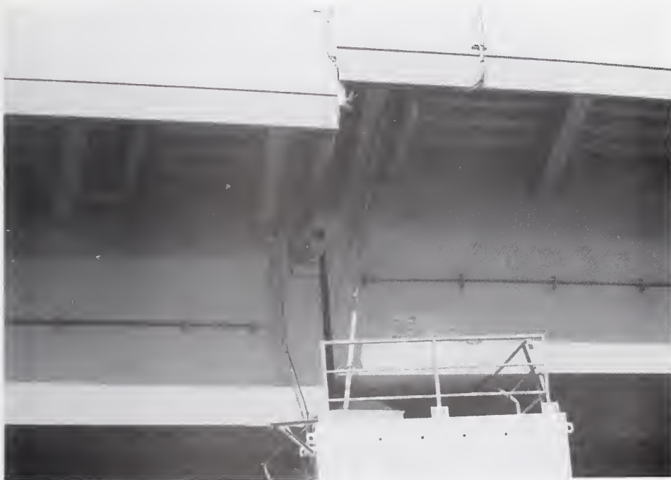
Figure 4.2.44 Approach span at edge of seat at Pier 134 of Shukugawa Bridge due to lateral movement of the pier by about 1 m towards the center of the channel.
