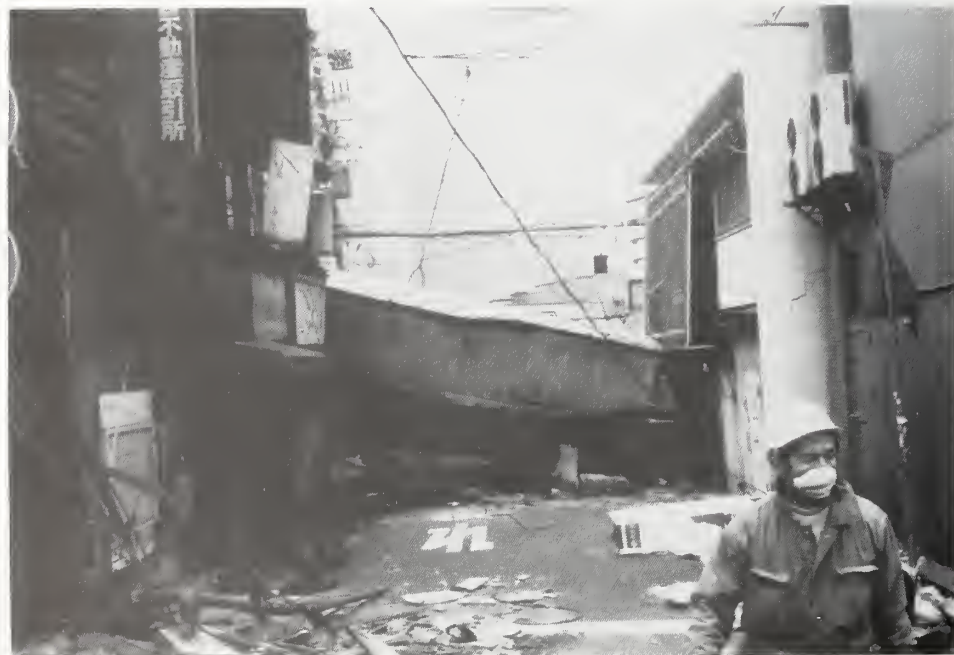
Figure 6.2.24 Road blocked by collapsed structure.
