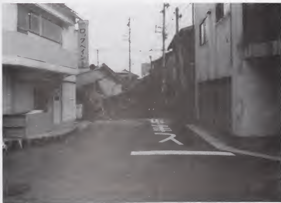
Figure 6.2.10 Collapsed structure across street.
