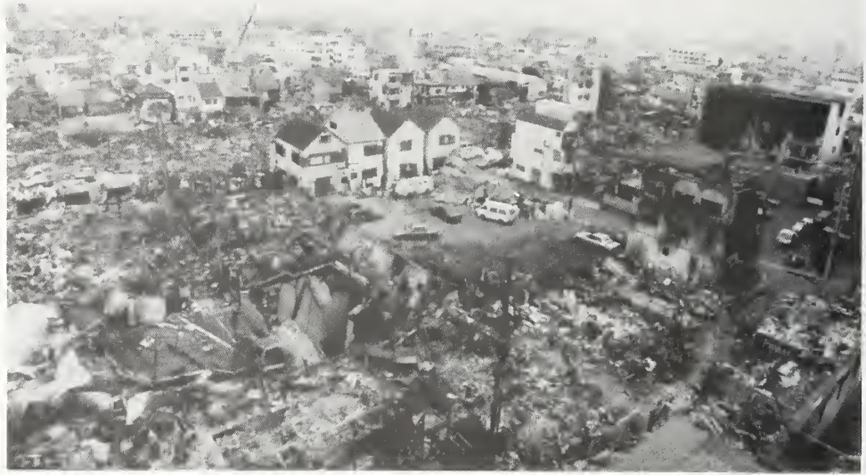
Figure 6.2.3 View of post earthquake fire damage in Nada Ward, Kobe (Site No. 8).
