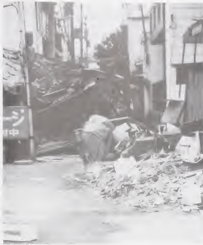
Figure 6.2.25 Road blocked by collapsed structure.
