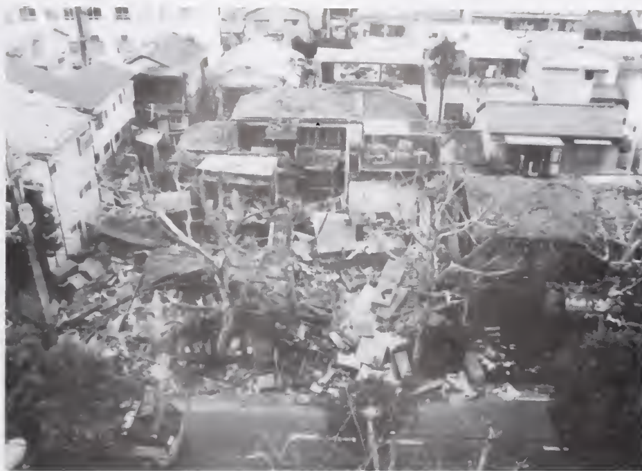
Figure 6.2.9 Collapsed houses. Notice that the pile of debris is in contact with the adjacent houses, forming a continuous fuel chain.
