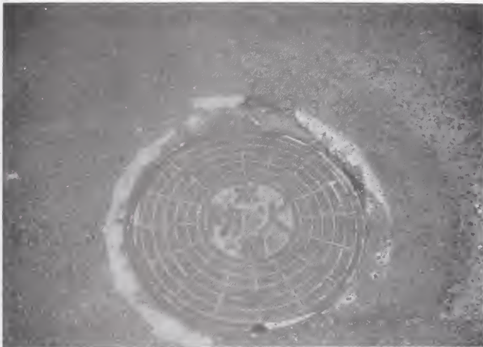
Figure 6.2.22 Access cover to unreinforced fire fighting water cistern .
