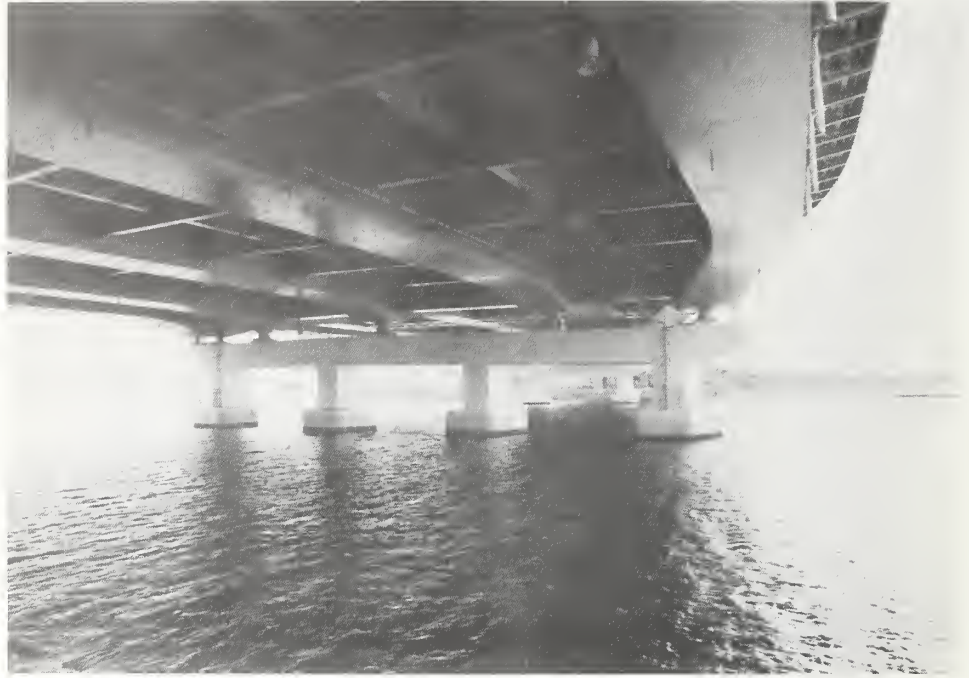
Figure 4.2.41 General view of the Shukugawa Bridge on Route 5.
