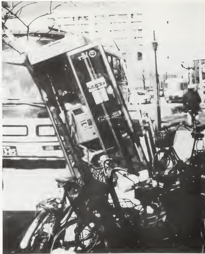
Figure 5.5.12 Soil instability damaged telephone booths.
