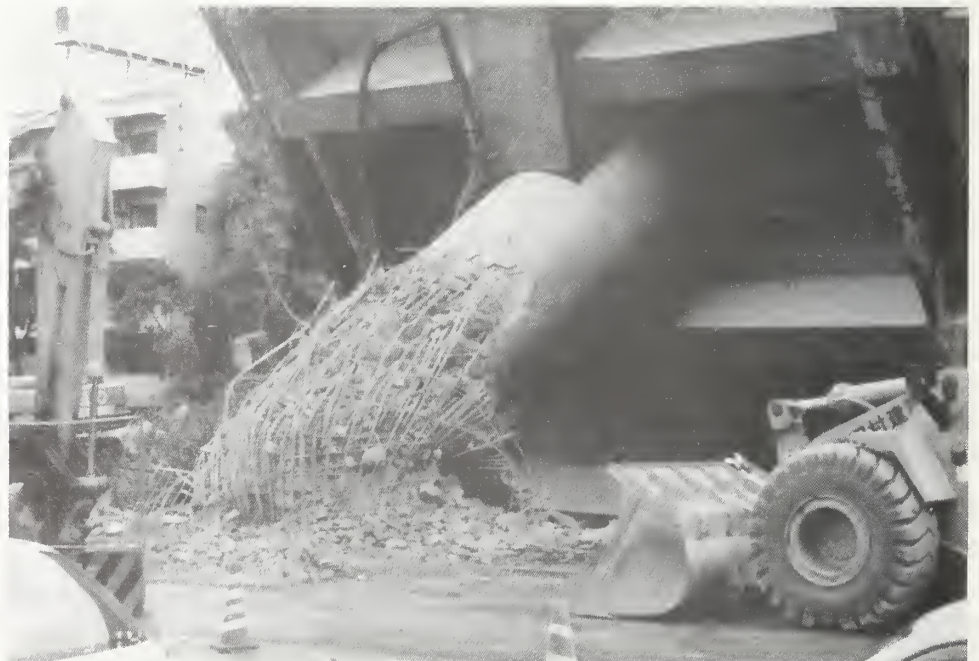
Figure 4.2.16 Higashi-Nada Viaduct, Pier 134.
