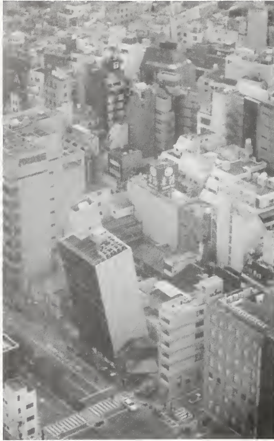
Figure 3.4.27 A leaning 9-story SRC building on Flower Road prior to total collapse.
