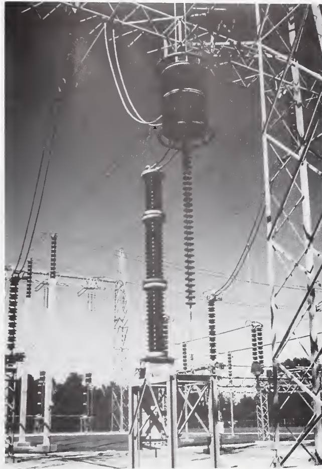
Figure 5.4.14 In the U.S. suspended wave traps usually have independent lower restraints
