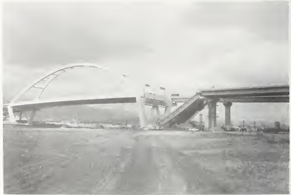
Figure 4.2.2a General view of Nishinomiya-ko Bridge, Route 5.
