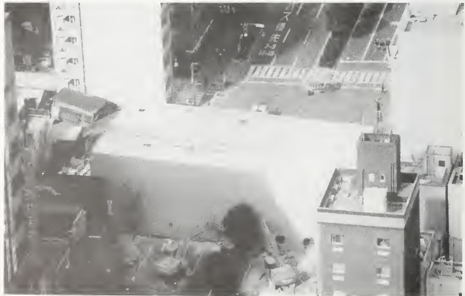
Figure 3.4.28 Totally collapsed building shown in Figure 3.4.27.
