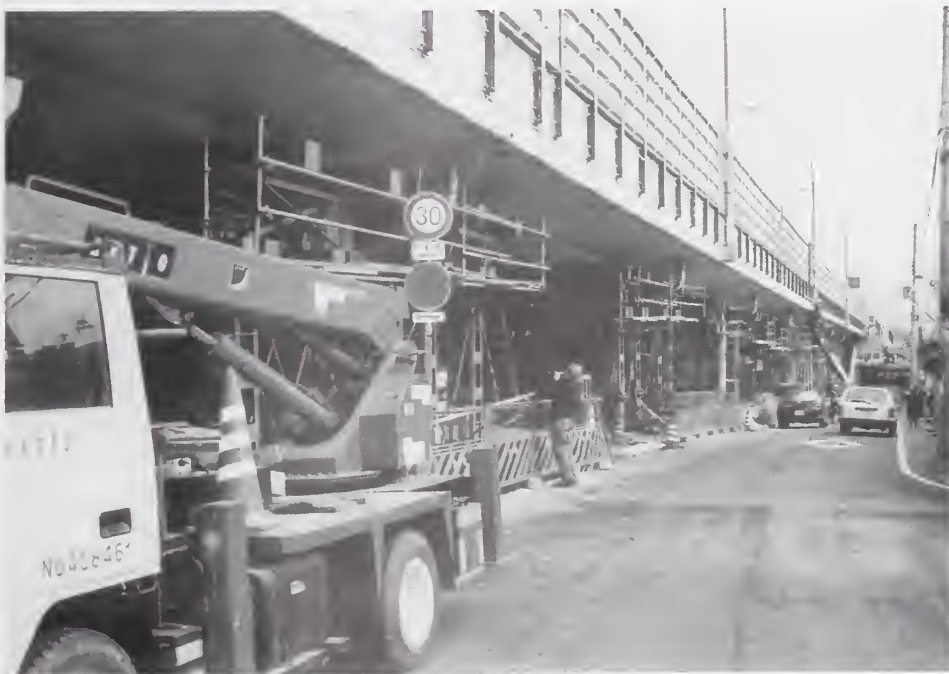
Figure 4.2.21 General view of Takarazuka Viaduct, Chugoku Expressway.
