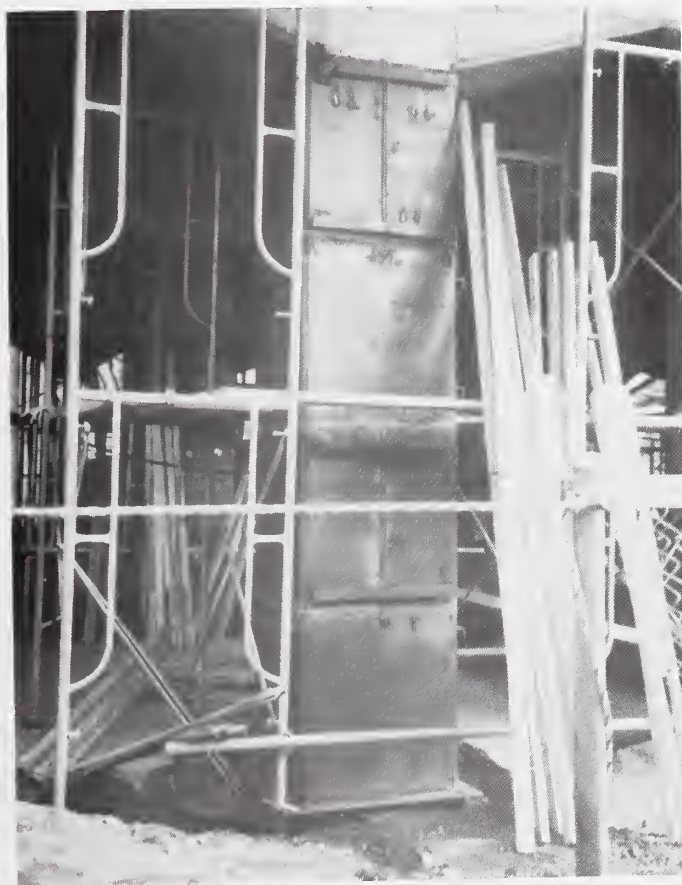
Figure 4.3.8 Jacketed column - JR Main Line.
