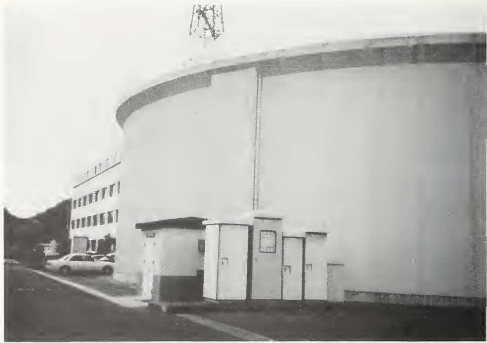
Photo 4 Concrete water storage tank at Okuhirano Purification Plant, less than 7 years old.
