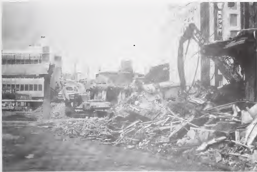
Figure 4.3.11 Collapsed Shin - Itami Station.
