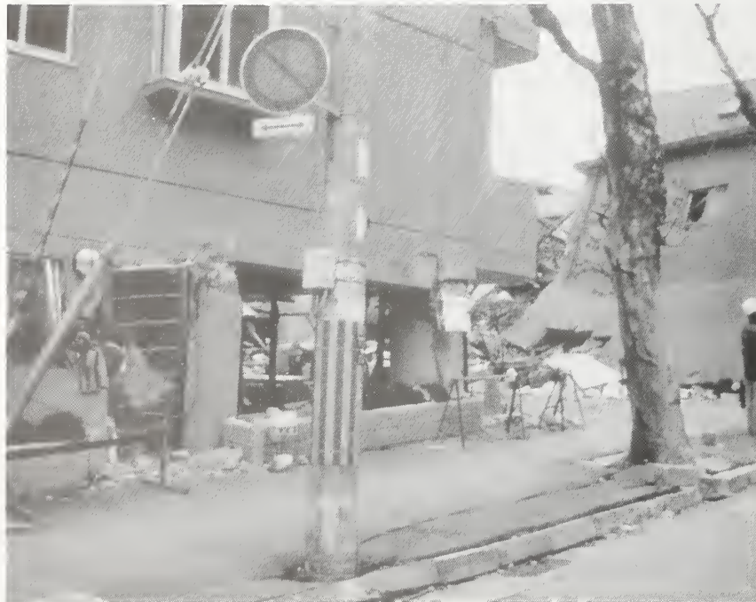
Figure 3.4.14 Collapsed first story near JR Line.
