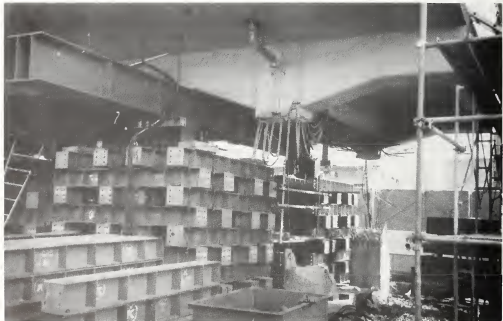
Figure 4.3.6 Column repair - Shinkansen.
