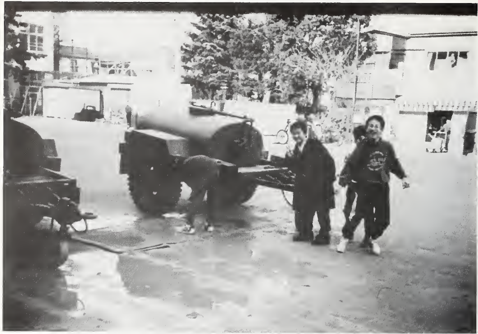
Photo 8 Emergency water supply delivered in tank trailer.
