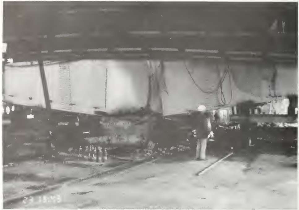
Figure 4.2.33 Pier 55, Route 3 near Tateishi.
