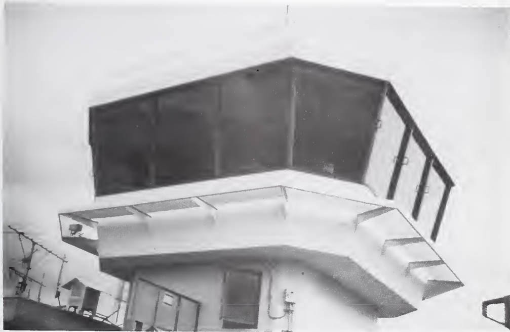
Figure 4.4.13 Cab of the Osaka Airport Control Tower.
