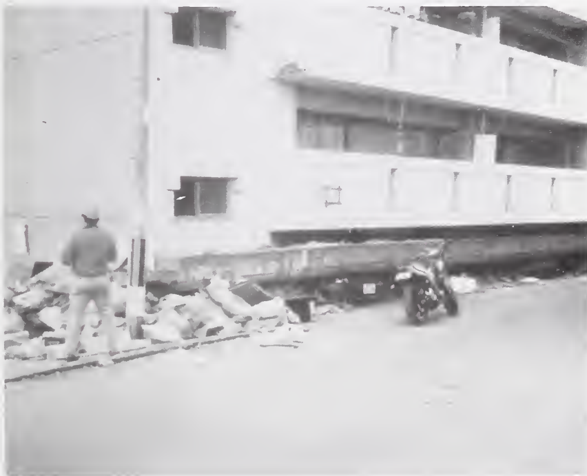
Figure 3.4.5 Failed ground floor shear wall - apartment building.
