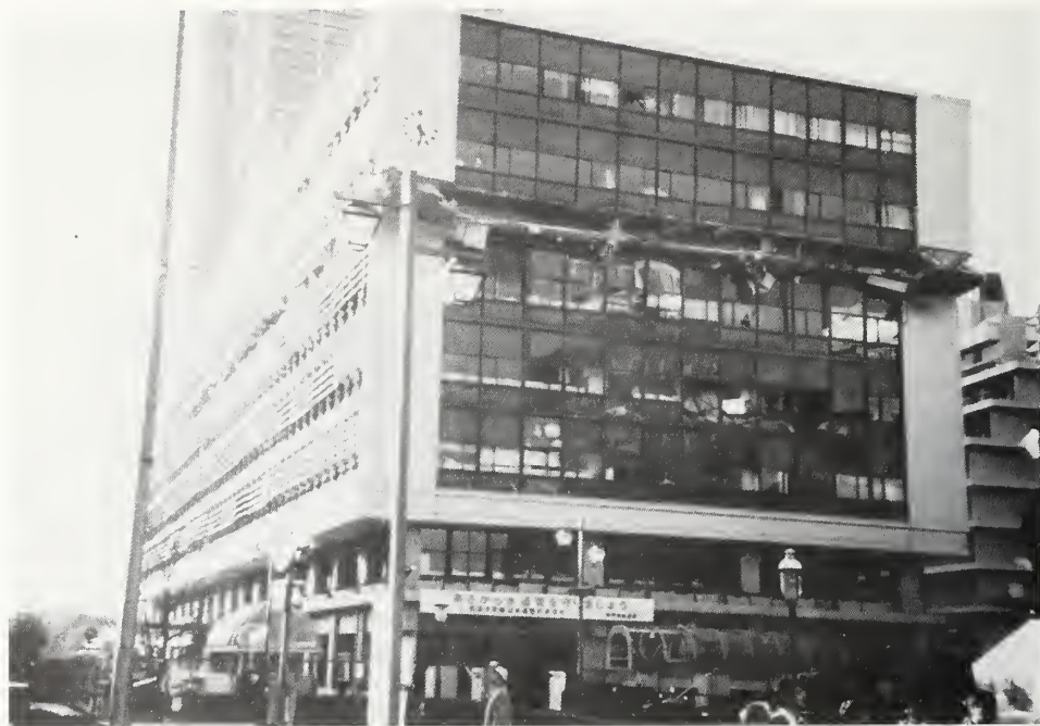
Photo 24 Pancaked sixth floor of City Hall Annex.
