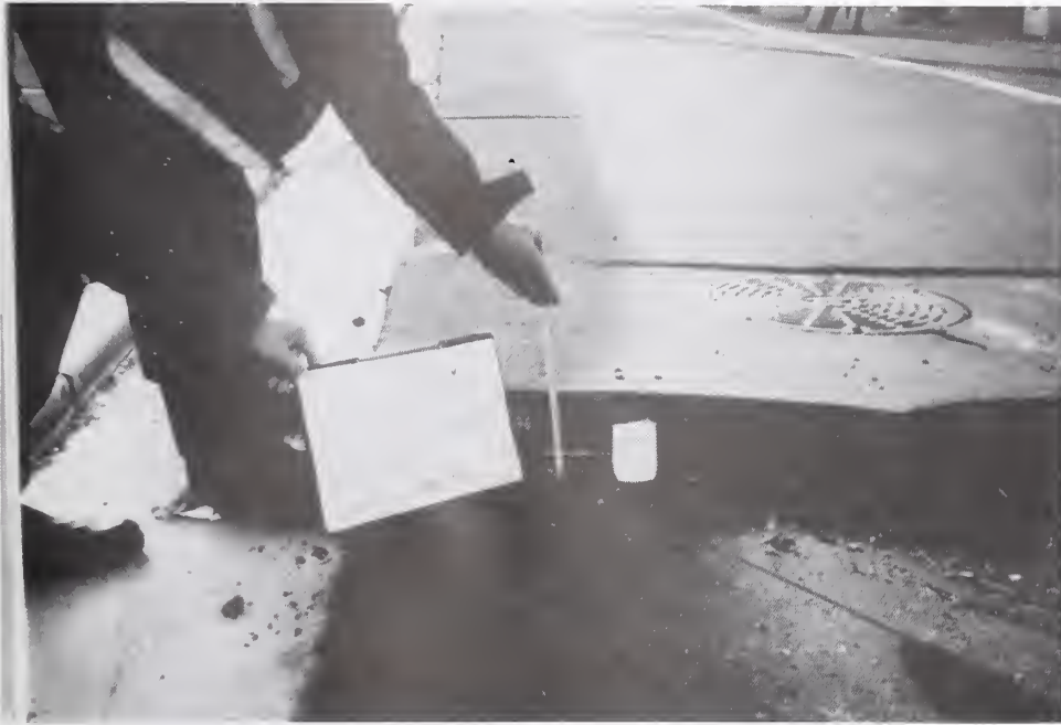
Figure 5.5.10 Large differential settlements in roadways can damage conduit and trunk lines.
