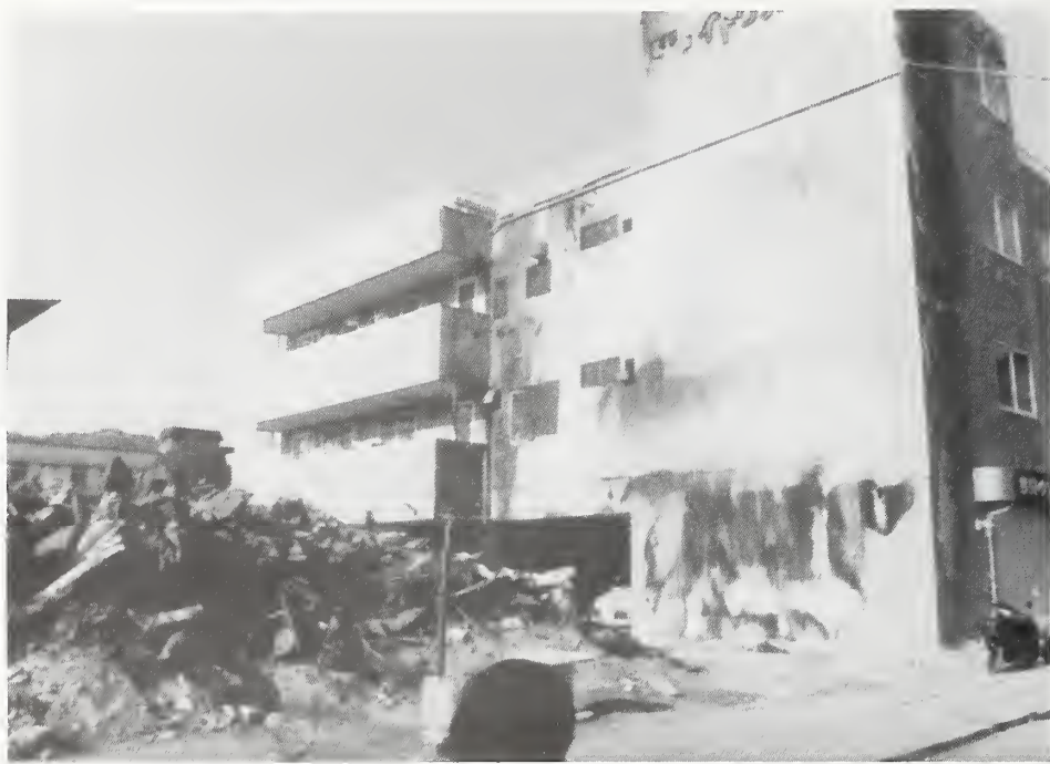
Figure 6.2.20 A building with a fire resistive exterior and wired glass windows.
