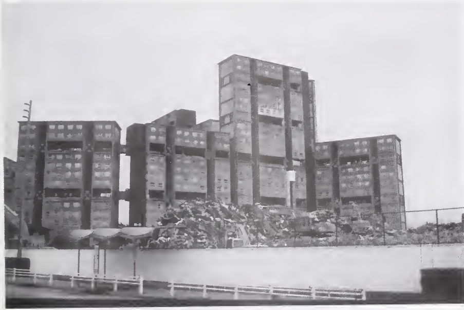
Figure 3.5.39 "Ashiya Hama Seaside Town" apartment complex.
