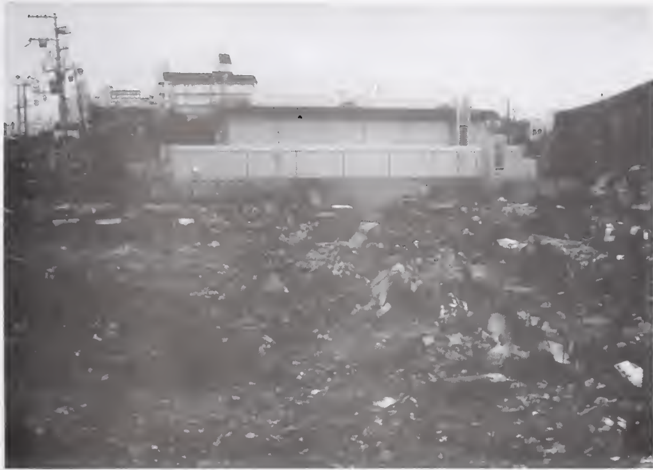
Figure 6.2.17 Electric Power Sub-Station.
