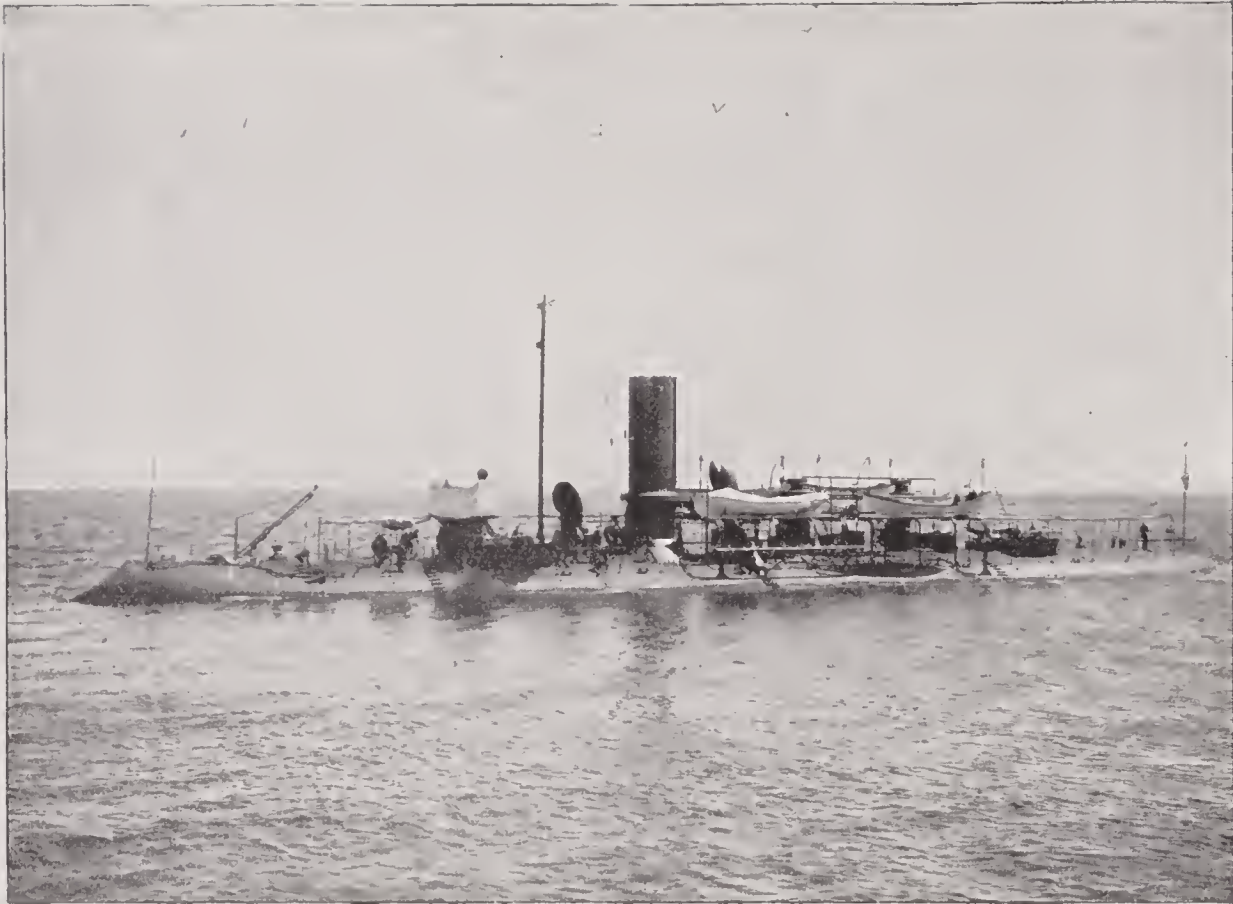
KATAHDIN —Twin-screw, steel, harbor-defense ram; 2,155 tons displacement; length, 250 feet 9 inches; breadth, 43 feet 5 inches; mean draft, 15 feet; horse power, 4,800; armor, 6 inches thick; batteries, four 6-pounder rapid-fire guns; speed, 17 knots an hour; crew, 30 officers and 91 men; cost, $930,000.
