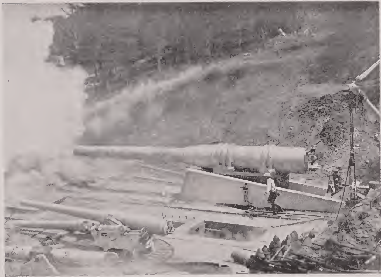
TWELVE-INCH BREECH-LOADING RIFLE —The photograph shows the gun mounted on shore for the purpose of testing. The weight of one shot from this weapon is 350 pounds. Guns of this description are built upon the principles of varying elasticity and initial tension, and are composed of a tube, jacket hoops, chase hoops and locking hoops.
