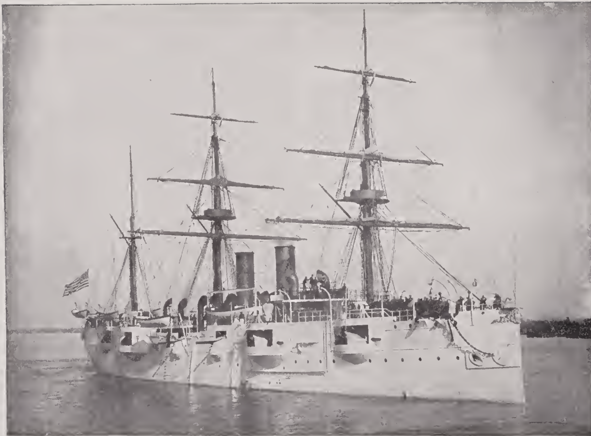
NEWARK —Steel, twin-screw, protected cruiser; 4,098 tons displacement; length, 310 feet; breadth, 49 feet 2 inches; mean draft, 18 feet 9 inches; horse power, 8,869; armament, main battery, twelve 6-inch breech-loading rifles; secondary battery, four 6 pounder rapid-fire guns, four 3-pounder rapid-fire cannons, four 37-millimetre Hotchkiss revolving cannons, and four Gatlings; speed, 19 knots an hour; crew, 34 officers and 350 men; cost, $1,379,897.47.
