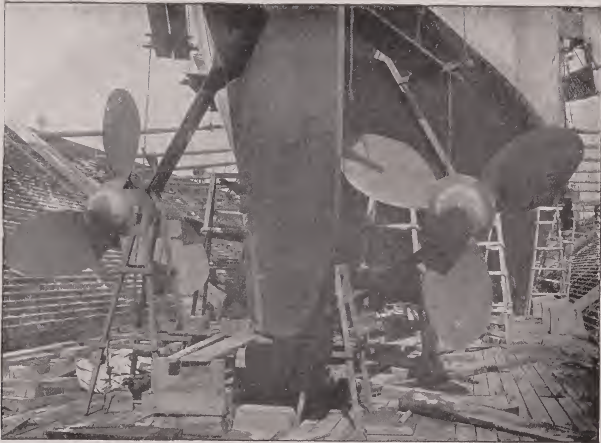
PROPELLERS OF THE NEW YORK —This photograph was taken specially to illustrate twin-screw propellers, which are the chief means of propulsion for most of the United States warships.
