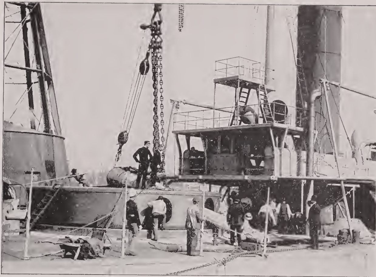
READY TO LOWER —The third of the series of photographs showing the process of placing large guns aboard a monitor. Having gotten the partly suspended gun at the correct angle the order is given to lower it to the sockets and rests prepared, when the greatest difficulty is overcome and the smaller details are proceeded with. In a very short time the cumbersome weapon is working with oily smoothness and fully prepared to spit defiance in the face of any and every enemy—excepting submarine mines.
