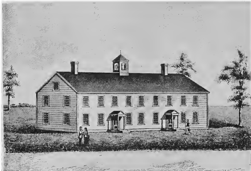
The Lopez House and Store, First Academy Building, 1784-1806, Leicester.
