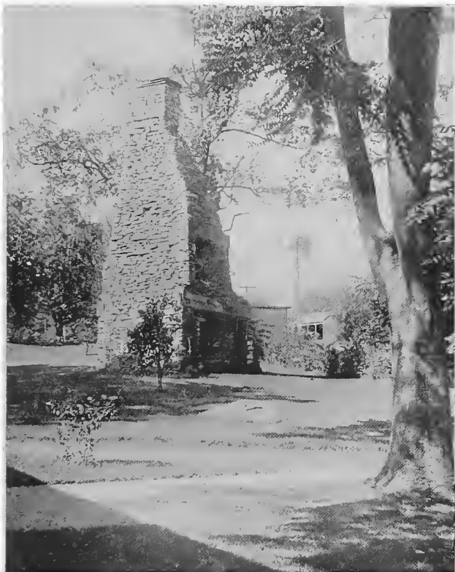
The Disbrow Chimney, Mamaroneck.
