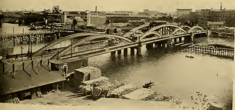
The Second Harlem, or Third Avenue Bridge. Made of Cast-iron, 1860.
