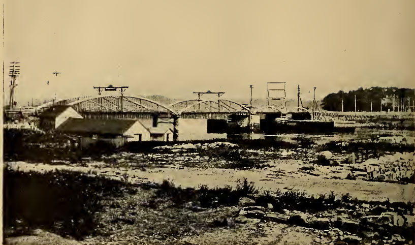
Pelham Bridge, over Eastchester Creek, Pelham Bay Park
