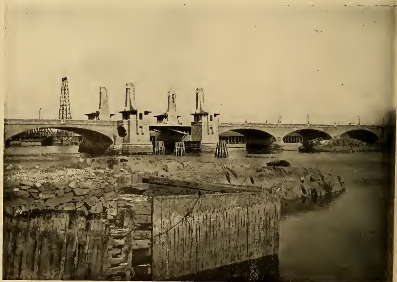
The New Pelham Bridge.
