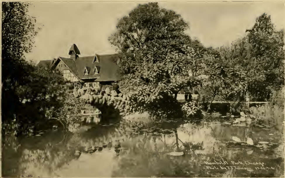
POLICE HEADQUARTERS, HUMBOLDT PARK
