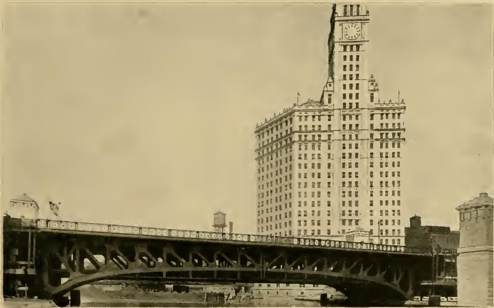
MICHIGAN BOULEVARD LINK BRIDGE
