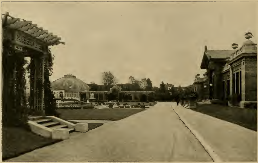
WASHINGTON PARK Administrative offices, conservatory, etc.
