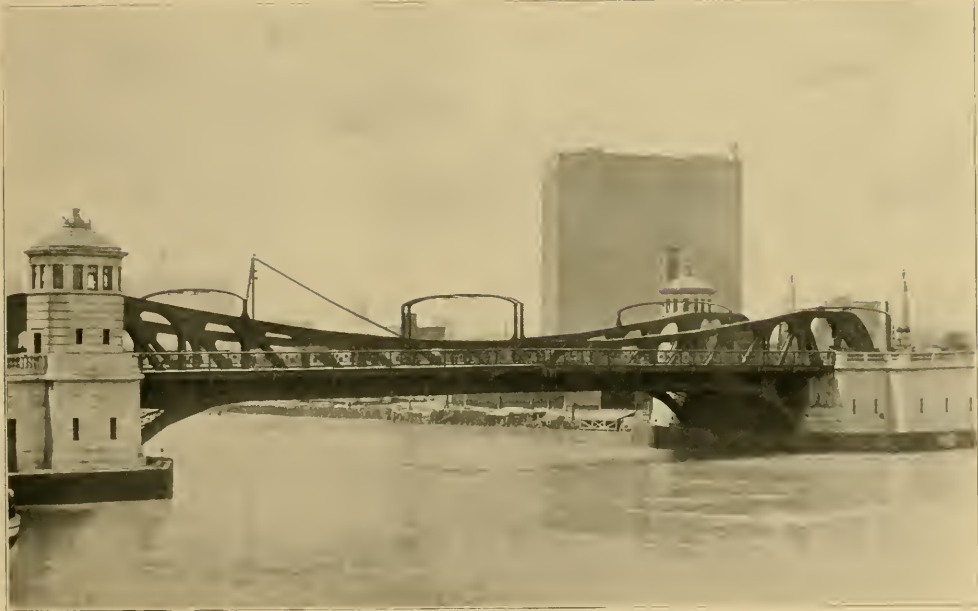
FRANKLIN - ORLEANS STREET LIFT BRIDGE Cost of bridge and approaches, $1,000,000.
