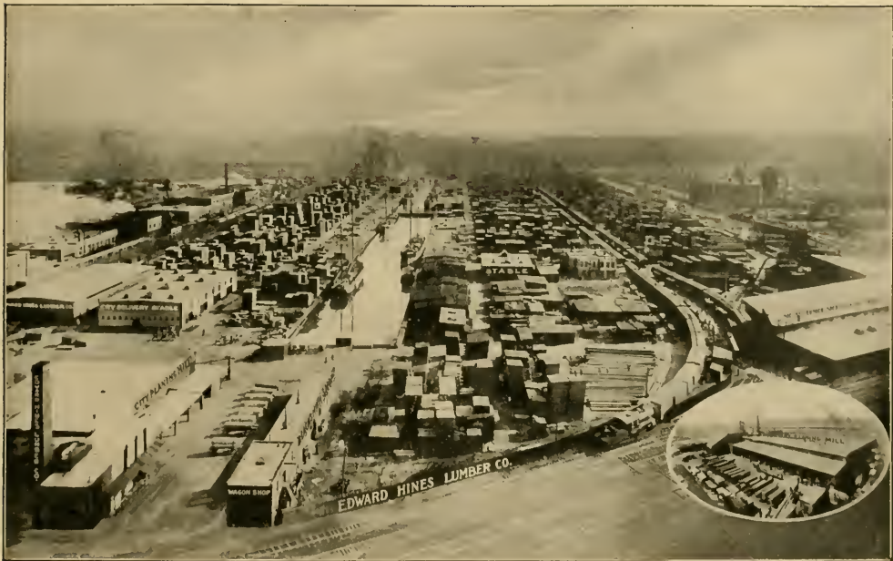
As viewed from tower 200 feet high, three large yards covering 45 acres, with water frontage of over a mile. The piling just opposite the locomotive, 1,000 in number and 60 feet long, gives an idea of the size of the plant
