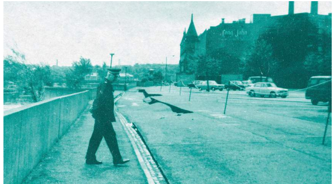
Above: Damage to the Gorbals riverbank caused by a weir failure in the 1970s. Photo by John Eadie
