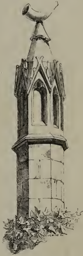
CHIMNEY, ST. BRIAVEL'S.
