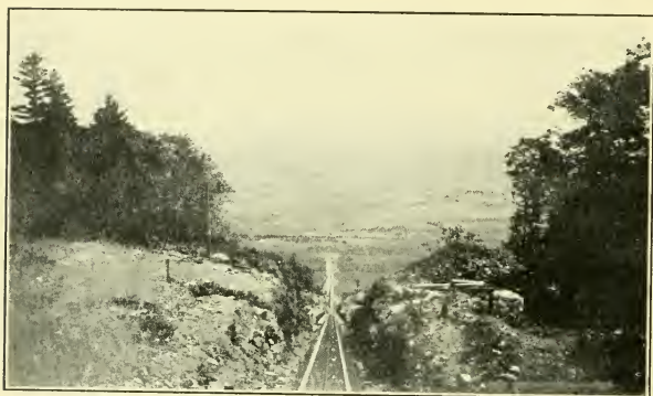
LOOKING DOWN THE OTIS ELEVATING RAILWAY EN ROUTE TO OTIS SUMMIT. HUDSON RIVER IN DISTANCE.
