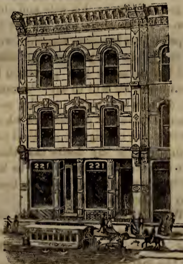
Front view of the CARPENTER DONATION, a fine, stone front building No. 221 West Madison St., Chicago, now occupied by the National Christian Association. The fee simple will be given by Mr. Carpenter if other friends raise $30,000 by Apr. 1st 1878, in cash or "good, negotiable, interest-bearing notes" to establish a Publishing House and headquarters of the reform. Send donations to the Treasurer at 18 Wabash Ave., Chicago.
