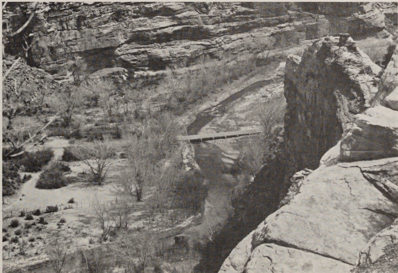
PHOTO 24 - State Route 12 crossing the Escalante River between Escalante and Boulder.
