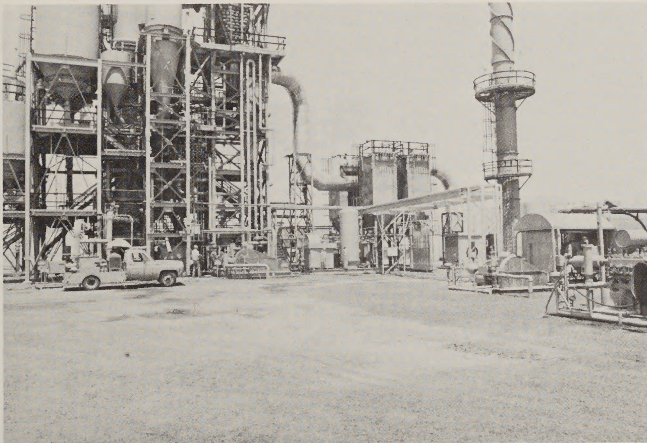
PHOTO 4 - Same facility as described above.
