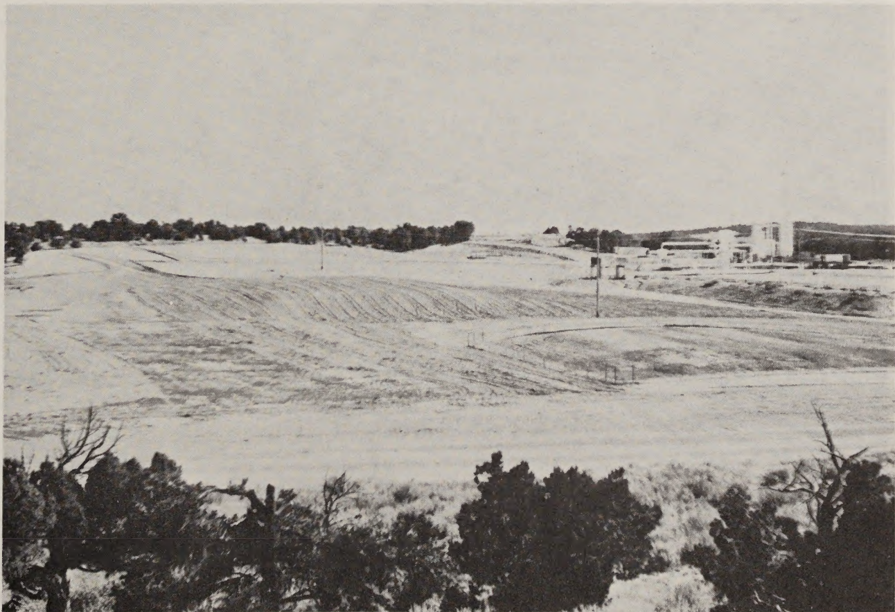
PHOTO 18 - Same area as shown in photo above.
