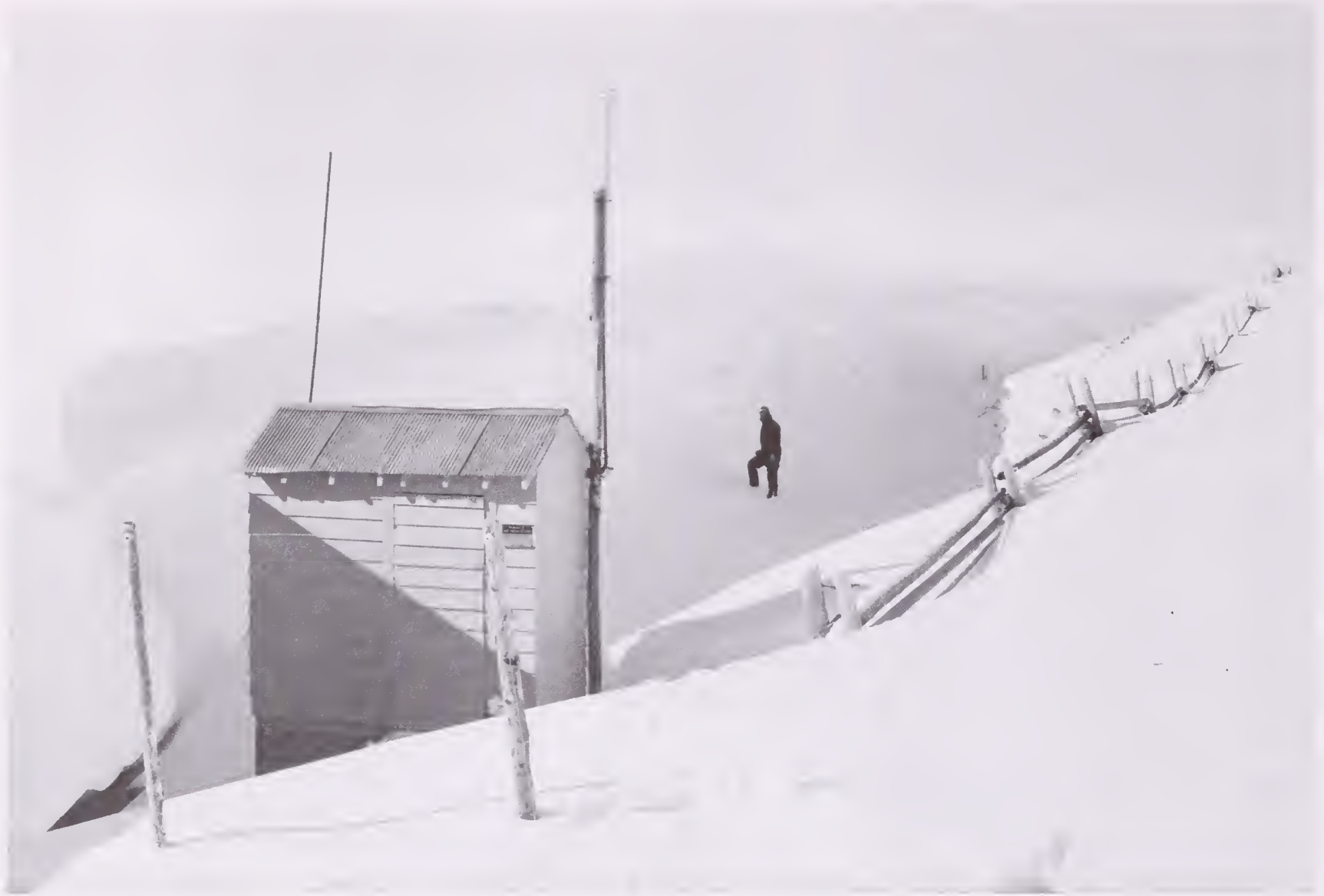
Figure 2b. — Appearance of the Sane Creek streamgage (February 26, 1980) in a normal winter at the time drifted snow covered the V-notch and stilling basin and was about to extend over the building housing the water level recorder and pumping sediment sampler.
