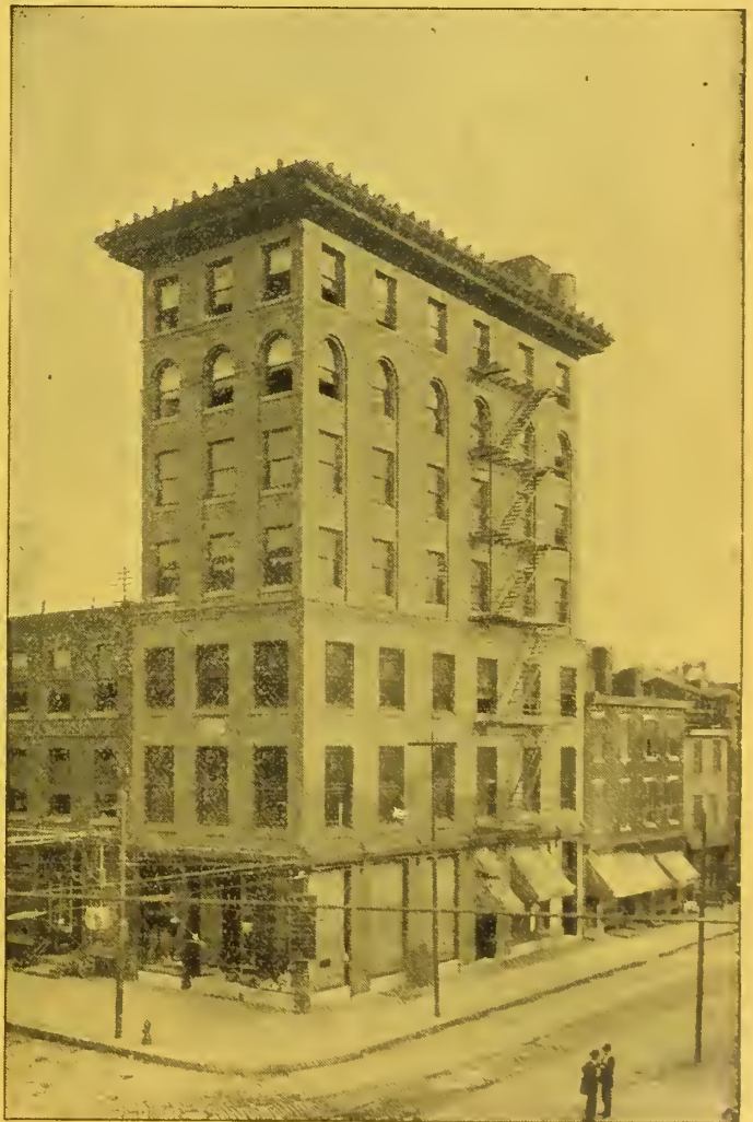
MAULE BUILDING, MARKET AND EIGHTEENTH STREETS
