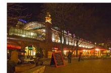
S-Bahn station Hackescher Markt
