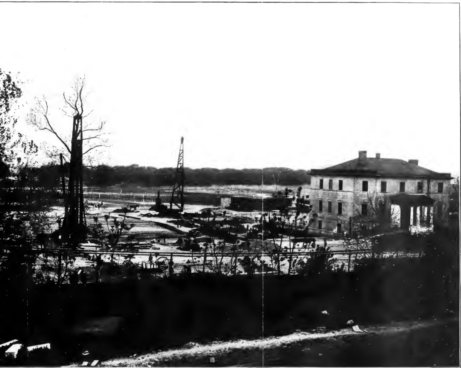
D SURROUNDINGS, SITE OF THE NEW BUILDING.
