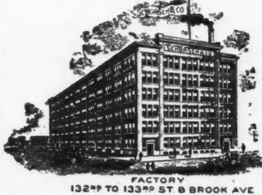
FACTORY 132 ND TO 133 RD ST & BROOK AVE
