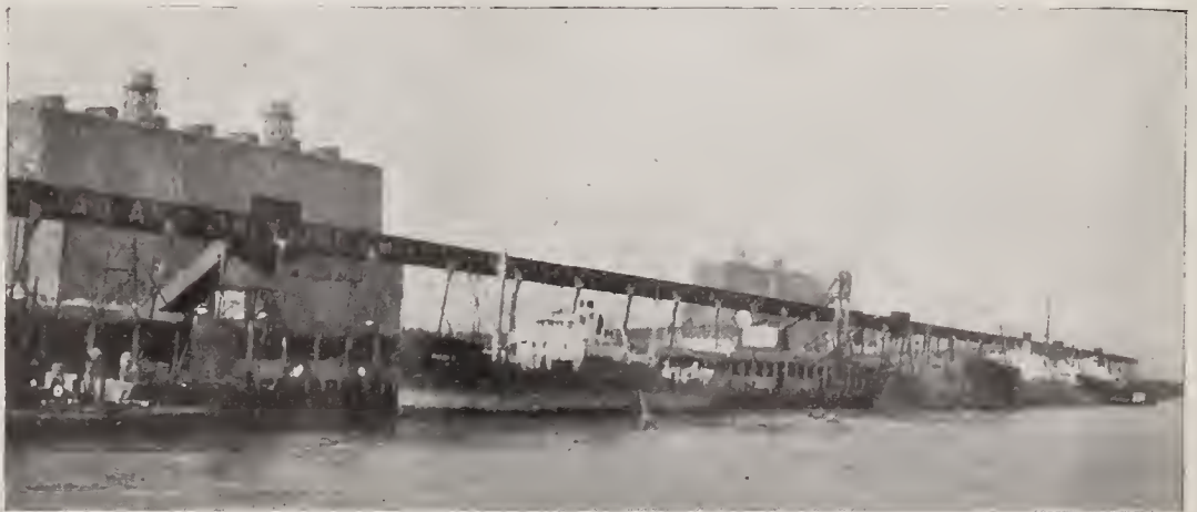
PARTIAL VIEW OF THE NEW ORLEANS WATERFRONT SHOWING I. C. ELEVATORS AND SECTION OF DOCKSIDE CONVEYOR GALLERY
