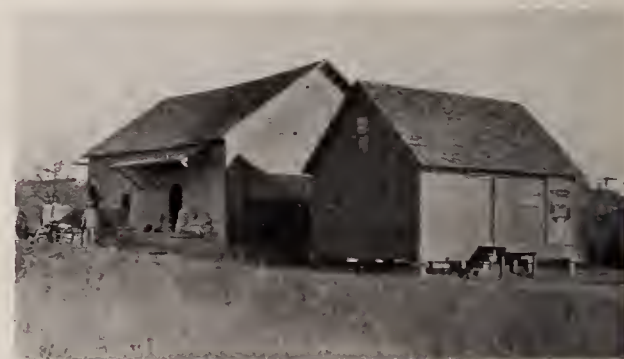
WAREHOUSE AND FEED MILL OF CHARLES H. EYLER
