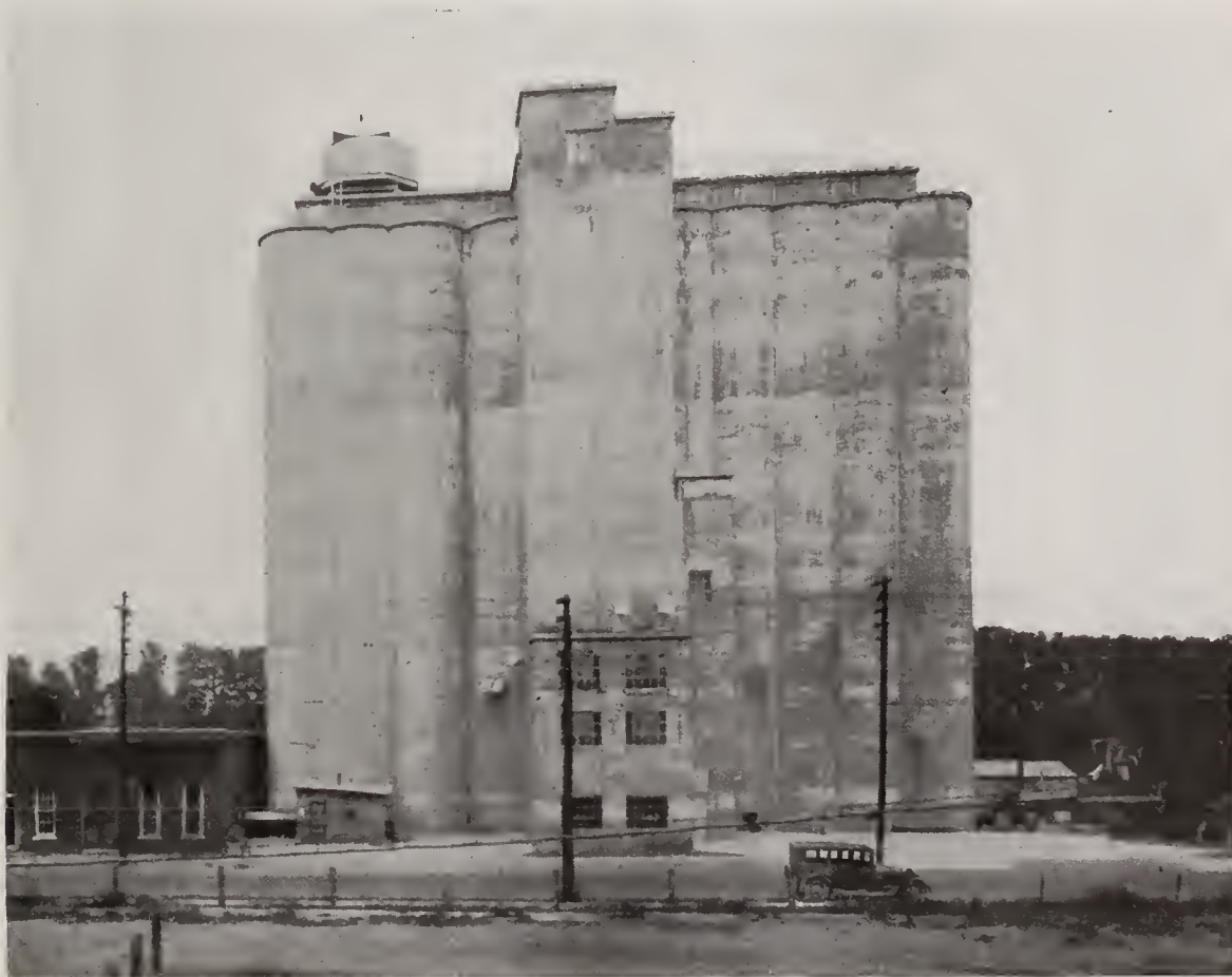
IGLEHEART BROS., INC., ELEVATOR, VINCENNES, IND.
