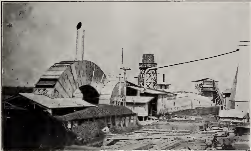
DEHYDRATING PLANT AT WARRINER MILL
