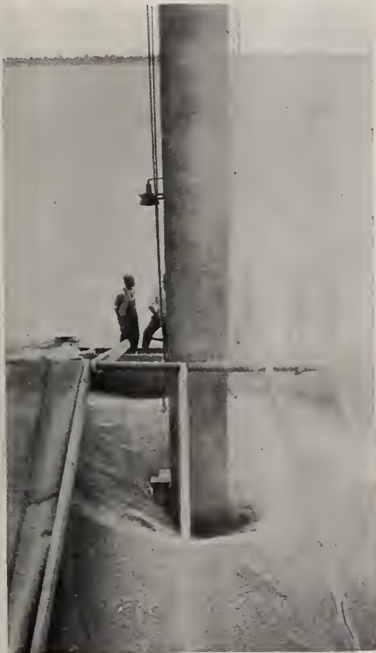
SUCTION LEG DRAWING GRAIN FROM BARGE TO NEW ORLEANS ELEVATOR BINS
