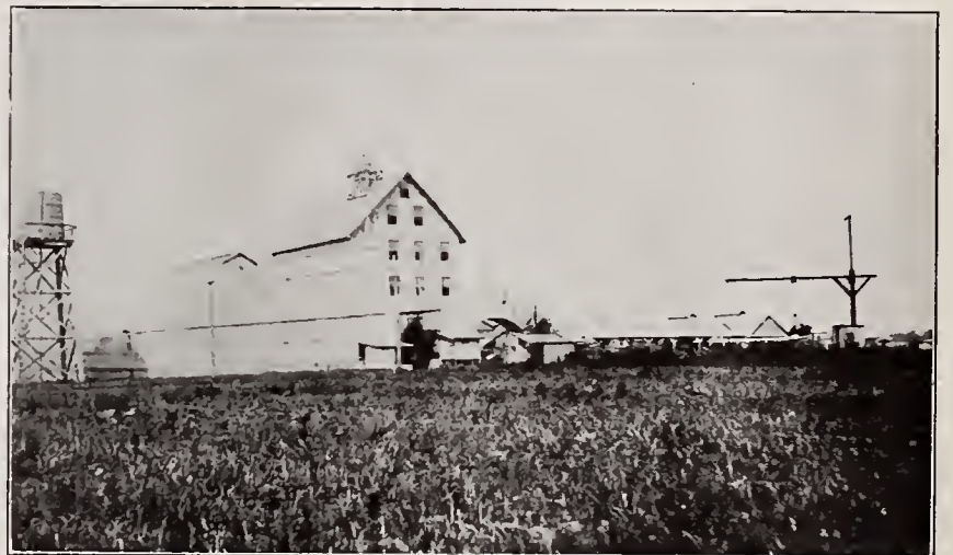
WARRINER FEED PLANT NEAR THIBODAUX
