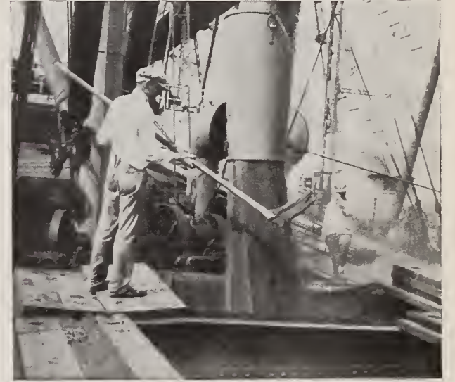
SAMPLING EUROPE-BOUND GRAIN WITH A PELICAN GRAIN TRIER
