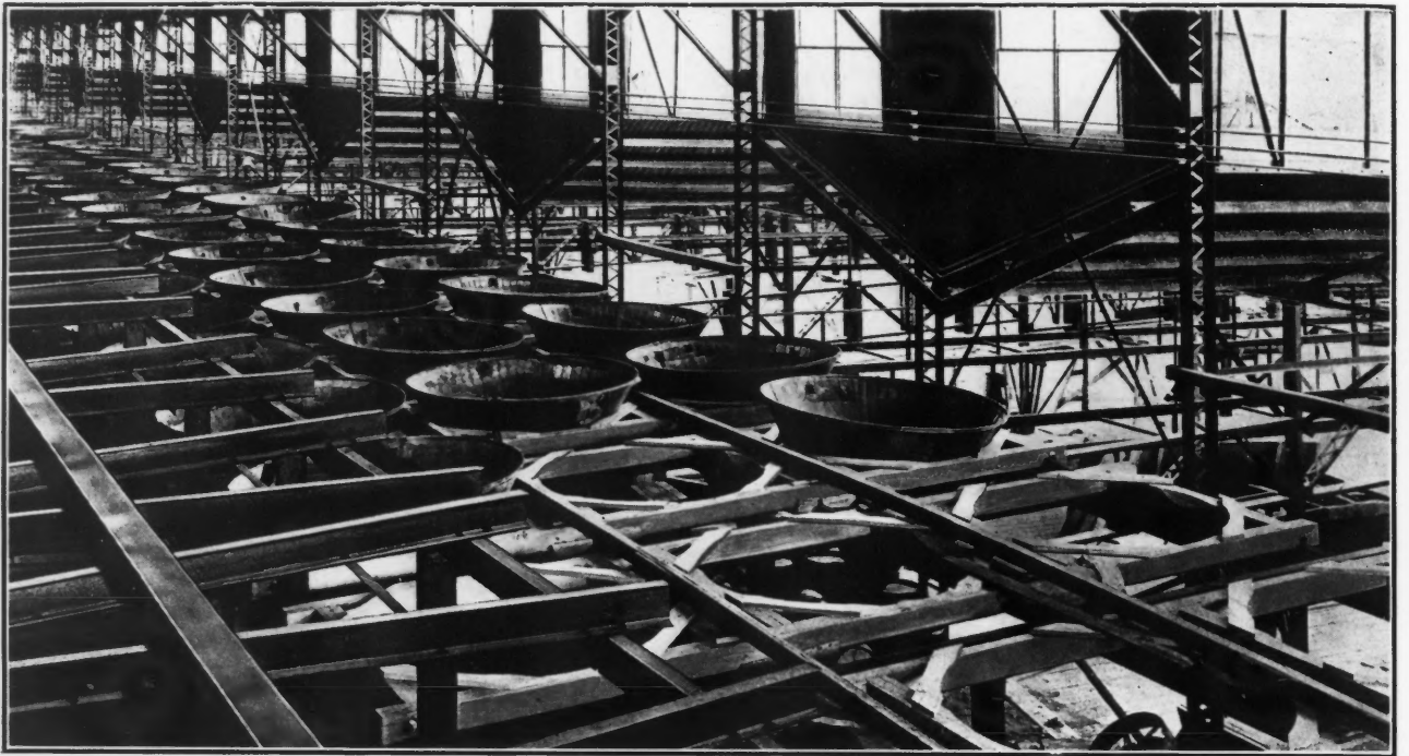
HYDRAULIC CLASSIFIERS, BOSTON MILL, GARFIELD, UTAH
