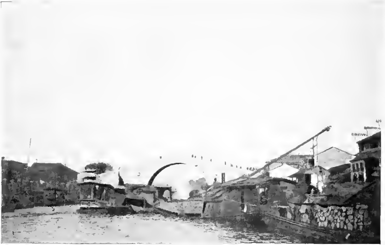
Bridge over Grand Canal at Wusih.
