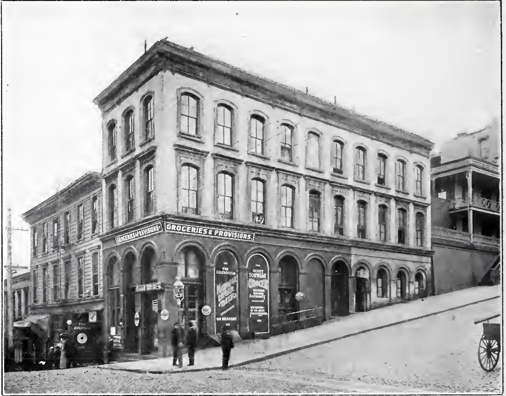
AN INTERESTING BASEMENT ARCADE.
