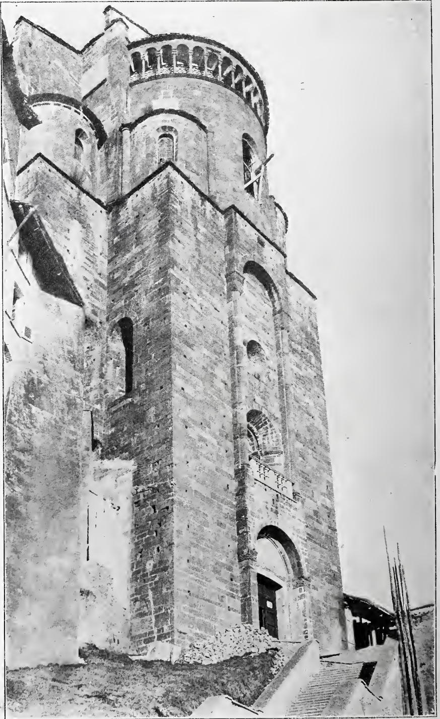
VIEW SHOWING THE MASSIVE WALLS SUPPORTING THE APSES OF THE SAGRA DE Piedmont, Italy. ST. MICHEL.
