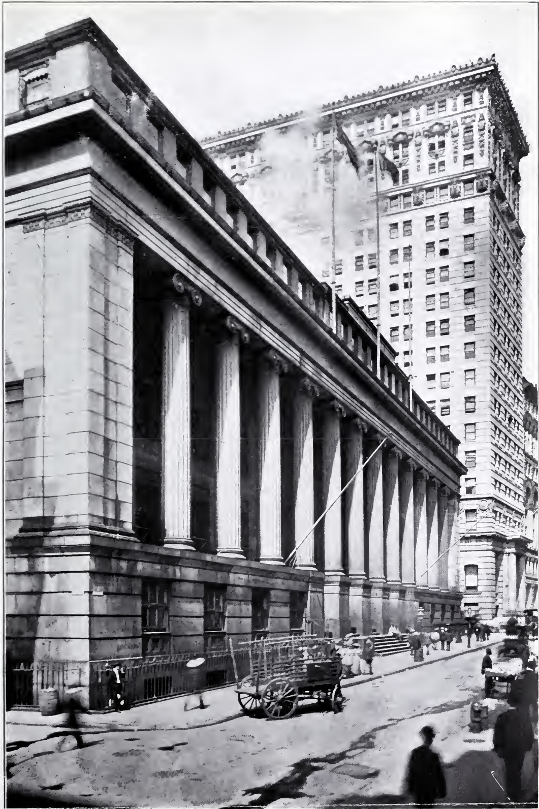
THE OLD CUSTOM HOUSE, NEW YORK.
