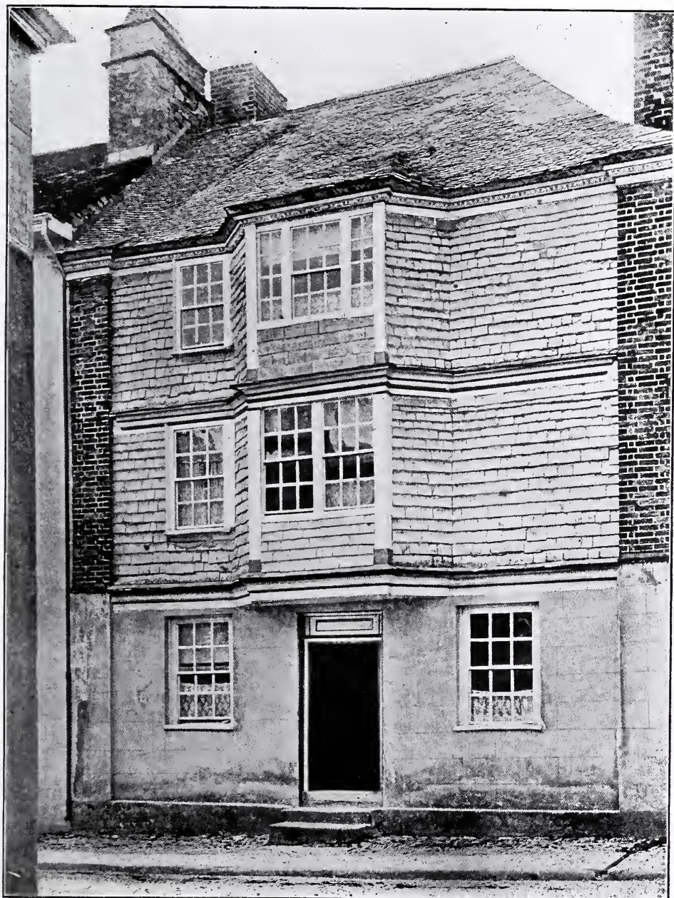
FIG. 10. HOUSE AT ASHBURTON. Slating replaces weather-boarding.
