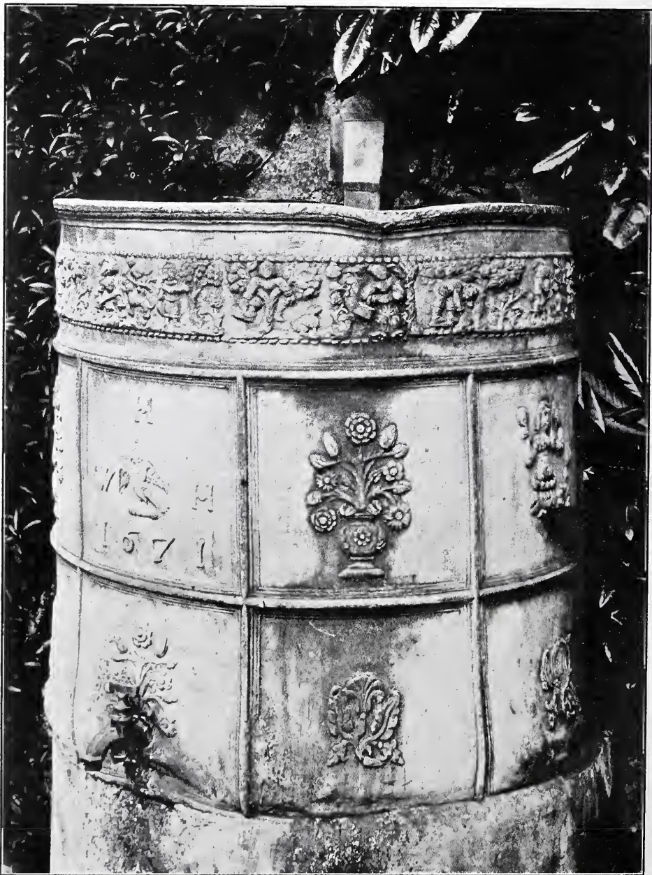
FIG. 11. CISTERN OF CAST LEAD, POUNDISFORD PARK, SOMERSETSHIRE.
