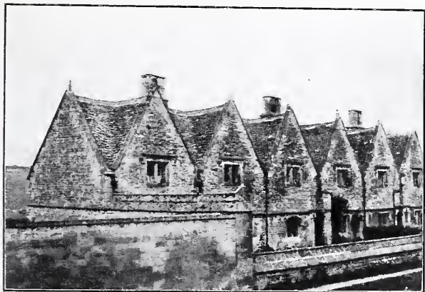
Fig. 7. Almshouse at Northleach. "Gables, a feature more noticeable in the stone districts."
