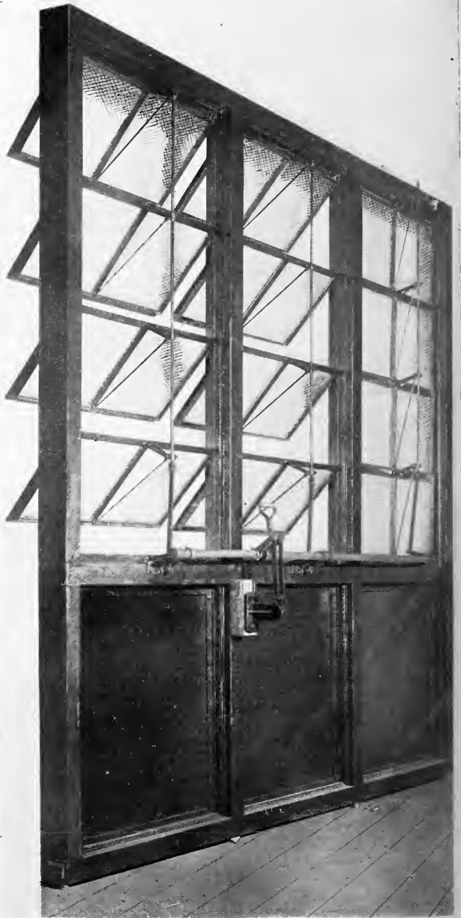
IRON AND WIRE GLASS WINDOW DETAIL—PENNSYLVANIA RAILROAD COMPANY'S NEW POWER HOUSE. Long Island City, N. Y. Westinghouse, Church, Kerr & Co., Engineers. The Hecla Iron Works, Contractors.
