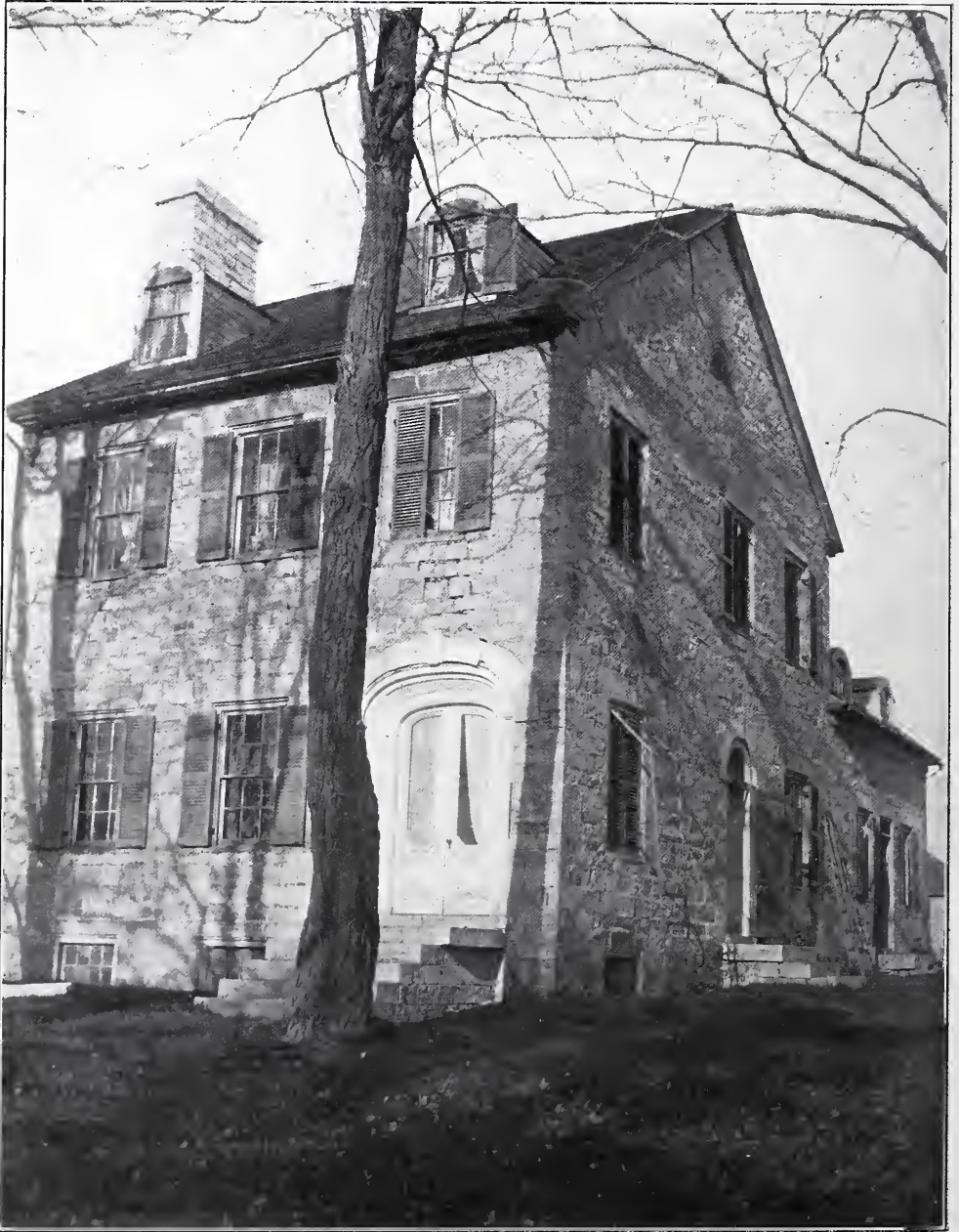
FIG. 10. A STONE HOUSE AT CHAUMONT, NEW YORK. (Built by Le Ray in 1820.)
