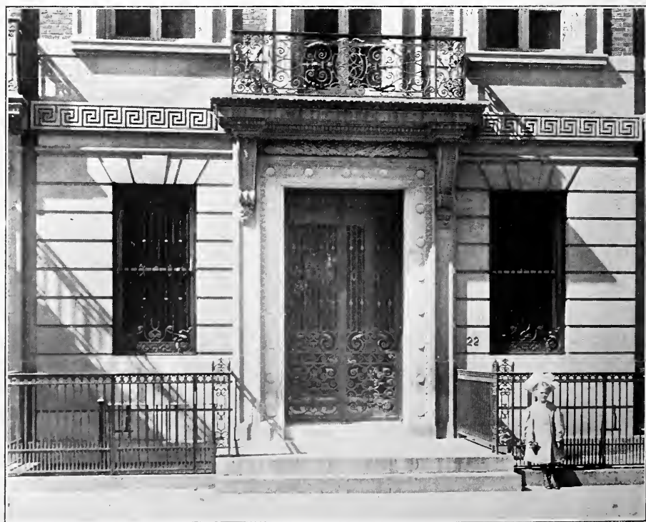
THE CLARK ESTATE HOUSES—DETAILS
