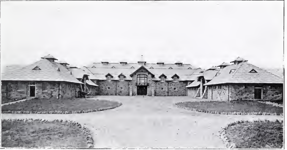
CONVERSE MANOR, THE ESTATE OF MR. E. C. CONVERSE.—THE STABLES. Greenwich, Conn. Donn Barber, Architect. (Photo by Alman & Co.)
