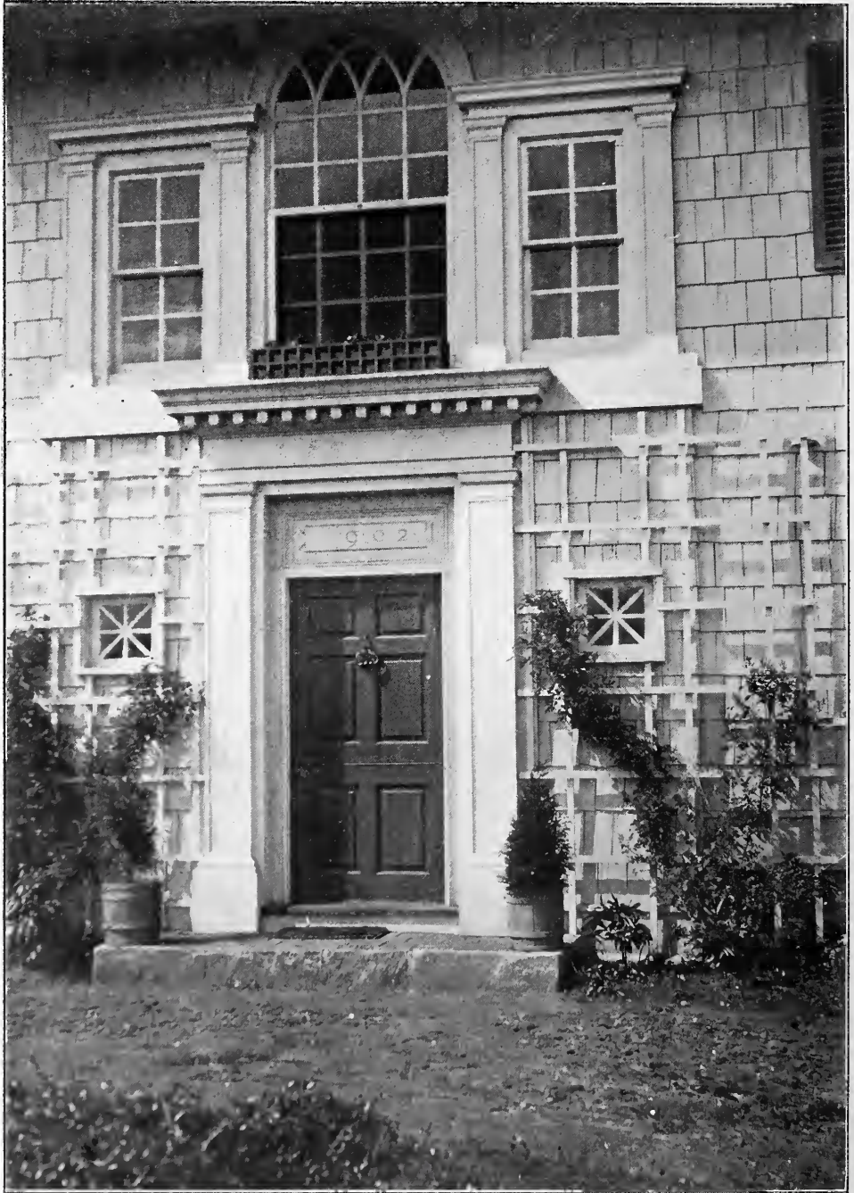
THE HOUSE OF F. C. CULVER, ESQ.—DETAIL OF ENTRANCE.
