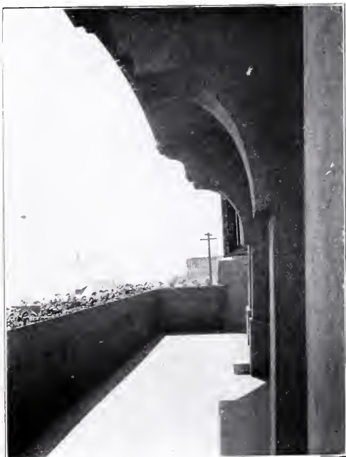
Fig. 6. A Detail of the Brackets of the East Porch.
