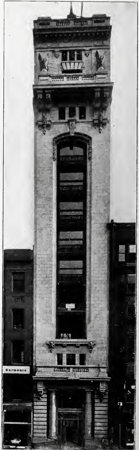
GUARDIAN SAVINGS AND TRUST CO. Cleveland, O. J. Milton Dyer, Architect.
