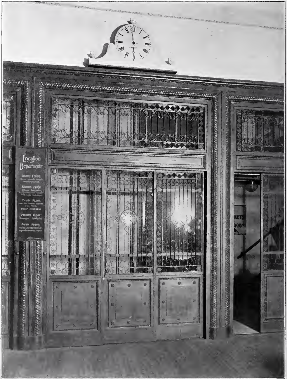
FIG. 6. A MORE ELABORATE METAL DECORATION WITH LESS GLASS SURFACE THAN FIG. 5. CHANDLER STORE BUILDING.
