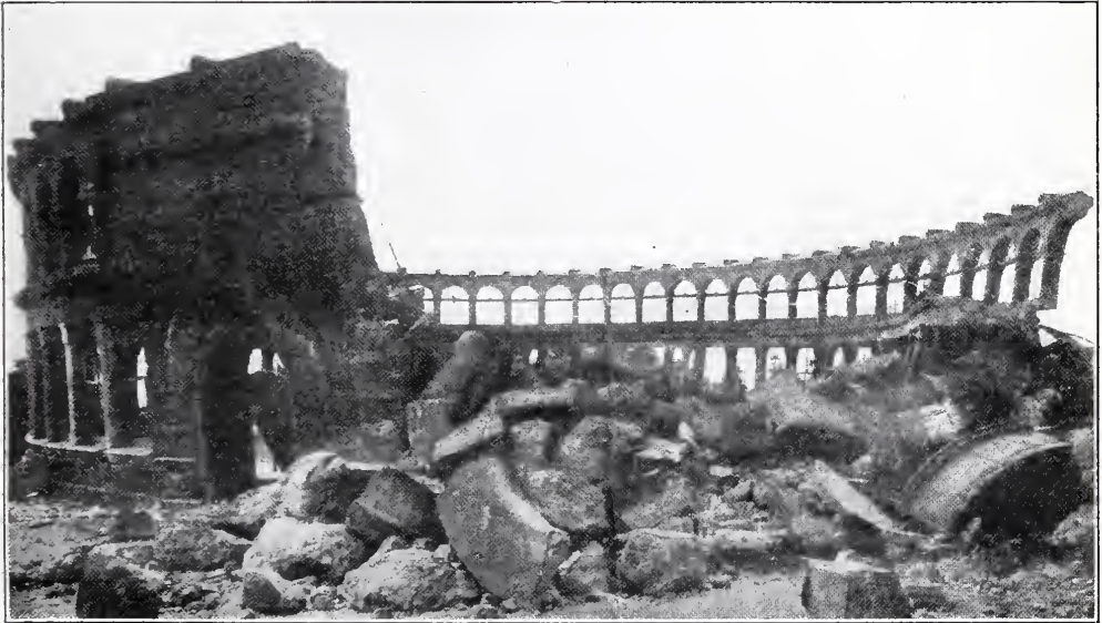
"THE PANORAMA," A CONCRETE STRUCTURE WRECKED BY THE EARTHQUAKE. Golden Gate Park, San Francisco, Cal.
