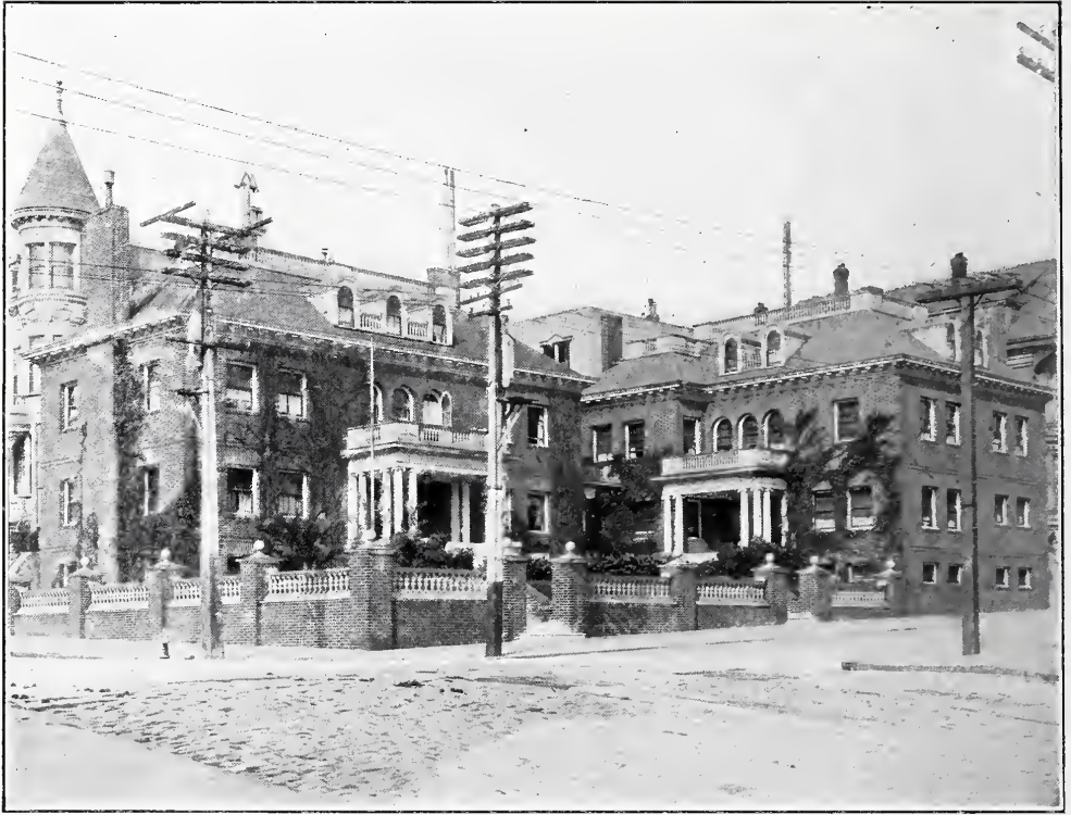
THE RESIDENCES OF MRS. SOPHIE LILIENTHAL AND MRS. BERTHA LILIENTHAL. San Francisco, Cal. Edgar A. Mathews, Architect.
