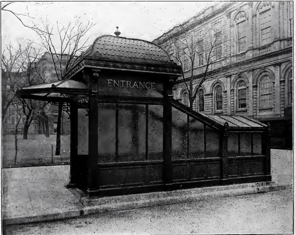
FIG. 9. A TYPICAL KIOSK OF THE INTERBOROUGH RAPID TRANSIT RAILROAD (SUBWAY). City Hall, N. Y. Heins & La Farge, Architects.
