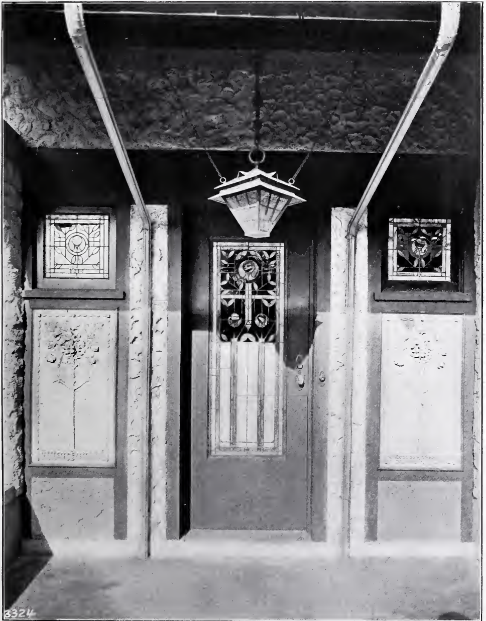
FIG. 3. A DETAIL OF THE PORCH SHOWN IN FIGS. 1 AND 2. MRS. WATERMAN'S HOUSE AT PARKERSBURG, WEST VIRGINIA.
