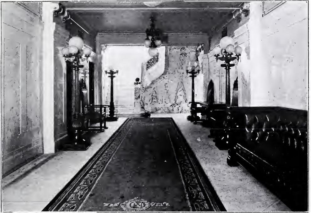
CENTRAL NATIONAL BANK—BASEMENT LOBBY.
