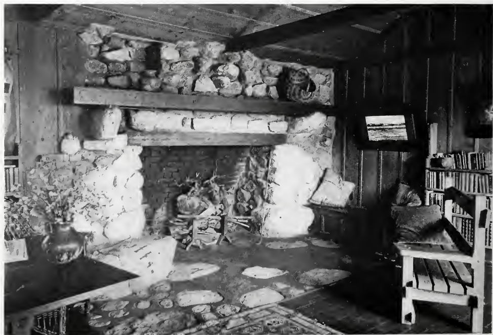
FIREPLACE IN THE LIVING-ROOM, MR. EDGAR A. CAMP'S HOUSE.
