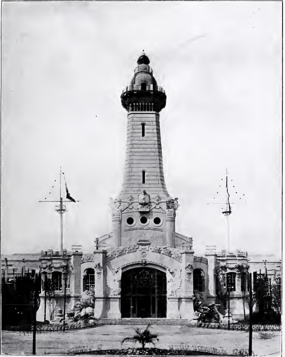
MARINE TRANSPORT, MAIN FRONT AND LIGHTHOUSE.
