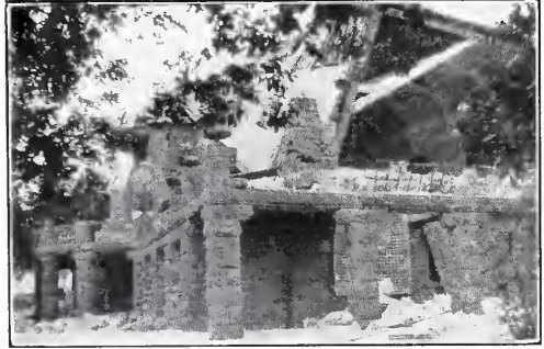
The "Children's Playhouse," Destroyed by the Earthquake. Golden Gate Park, San Francisco, Cal.
