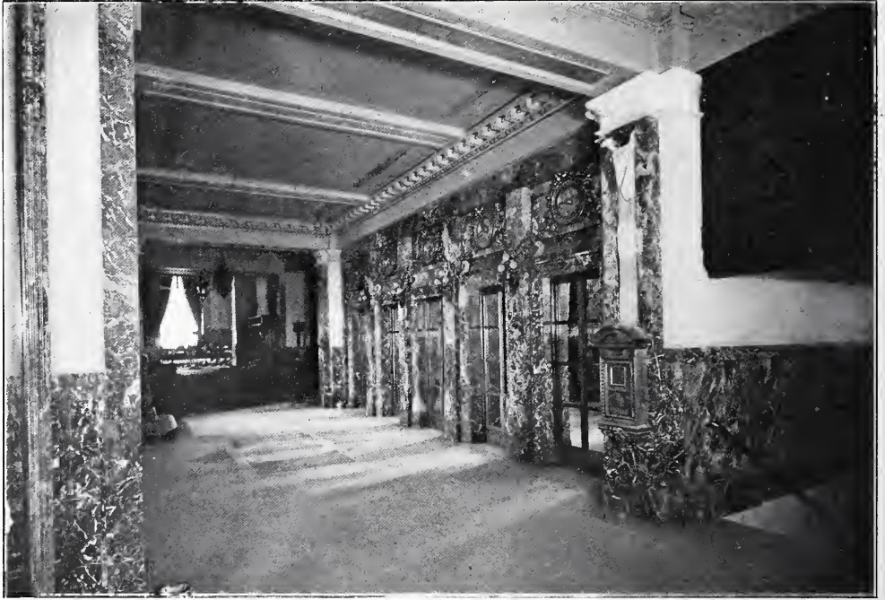
FIG. 5. THE ELEVATOR ENCLOSURES ARE TREATED IN MARBLE AND THE DOORS ARE COVERED WITH MIRRORS—HOTEL BELMONT.
