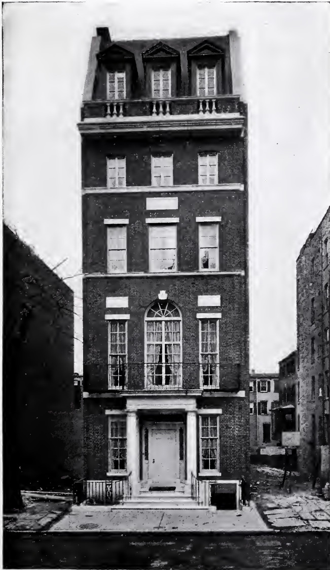
THE RESIDENCE OF CHARLES DANA GIBSON, ESQ. East 73d Street, New York.
