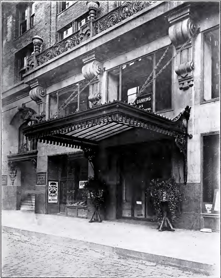
FIG. 7. A WELL-HUNG MARQUISE OF IRON AND WIRE GLASS. THE RECTOR BUILDING. Chicago, Ill. The Winslow Bros. Co., Manufacturers.
