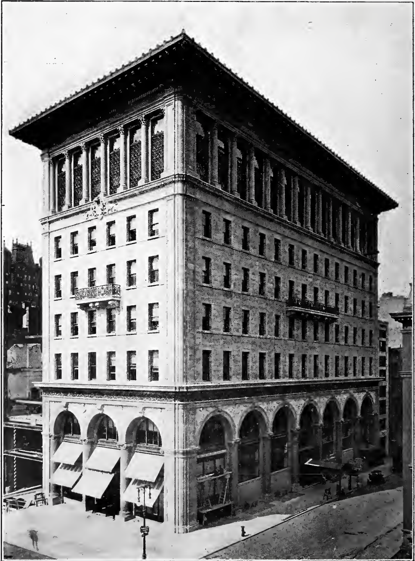
THE GORHAM MFG. CO'S BUILDING.
