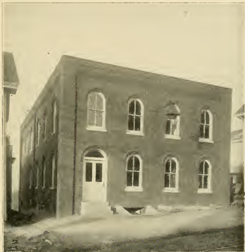
THE SUB-STATION ON PARK STREET
