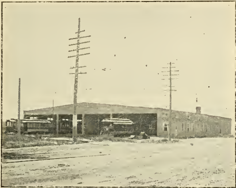
NEW CONCRETE CAR STABLE
