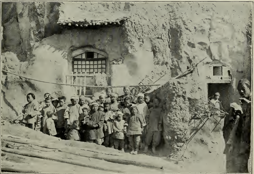
FIGURE 2.—HOUSE EXCAVATED IN LOESS AT SHIWANTSE HOUSES IN AND EROSIONS OF LOESS AT SHIWANTSE
