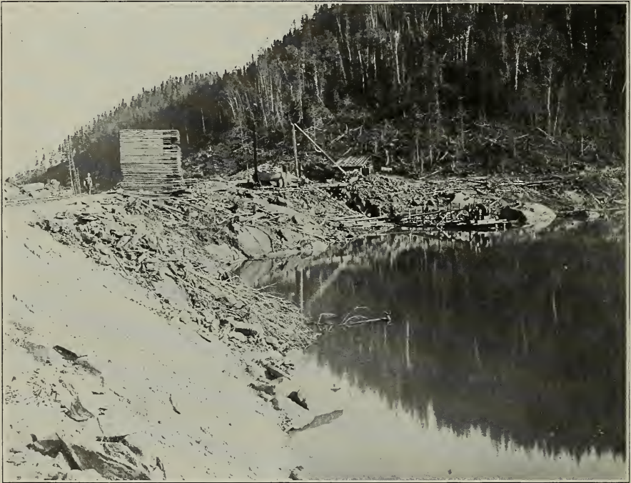
WEST END, BOYER LAKE, HELEN MINE
