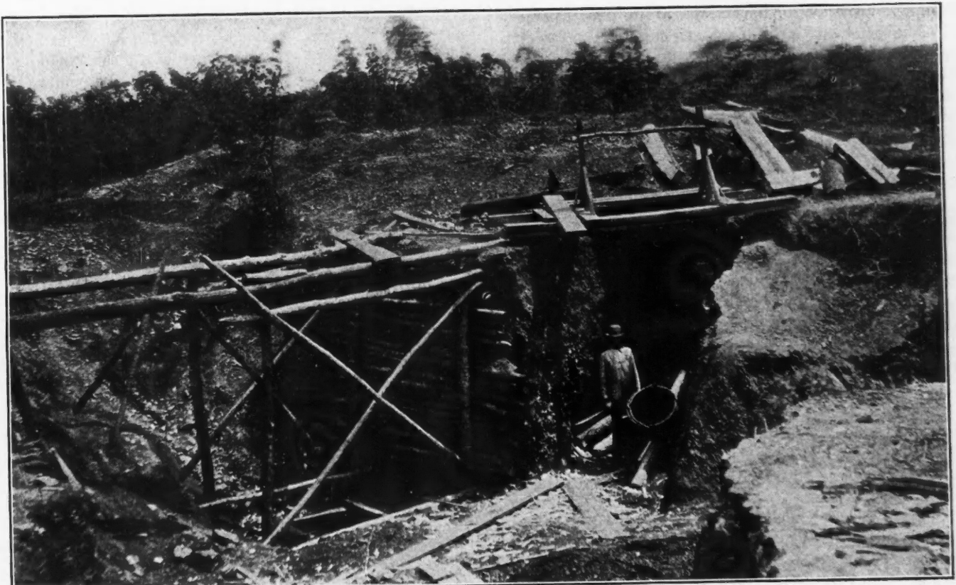
PIT, TUNNEL AND SHAFT WORKINGS OF BROOKS MINE, NEAR CUSHMAN
