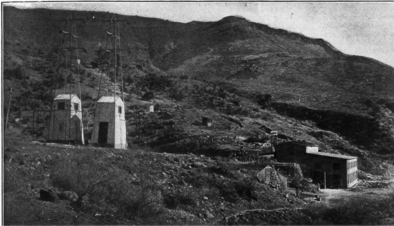
MAIN POWER PLANT OF ARIZONA POWER CO. ON VERDE RIVER, ARIZONA
