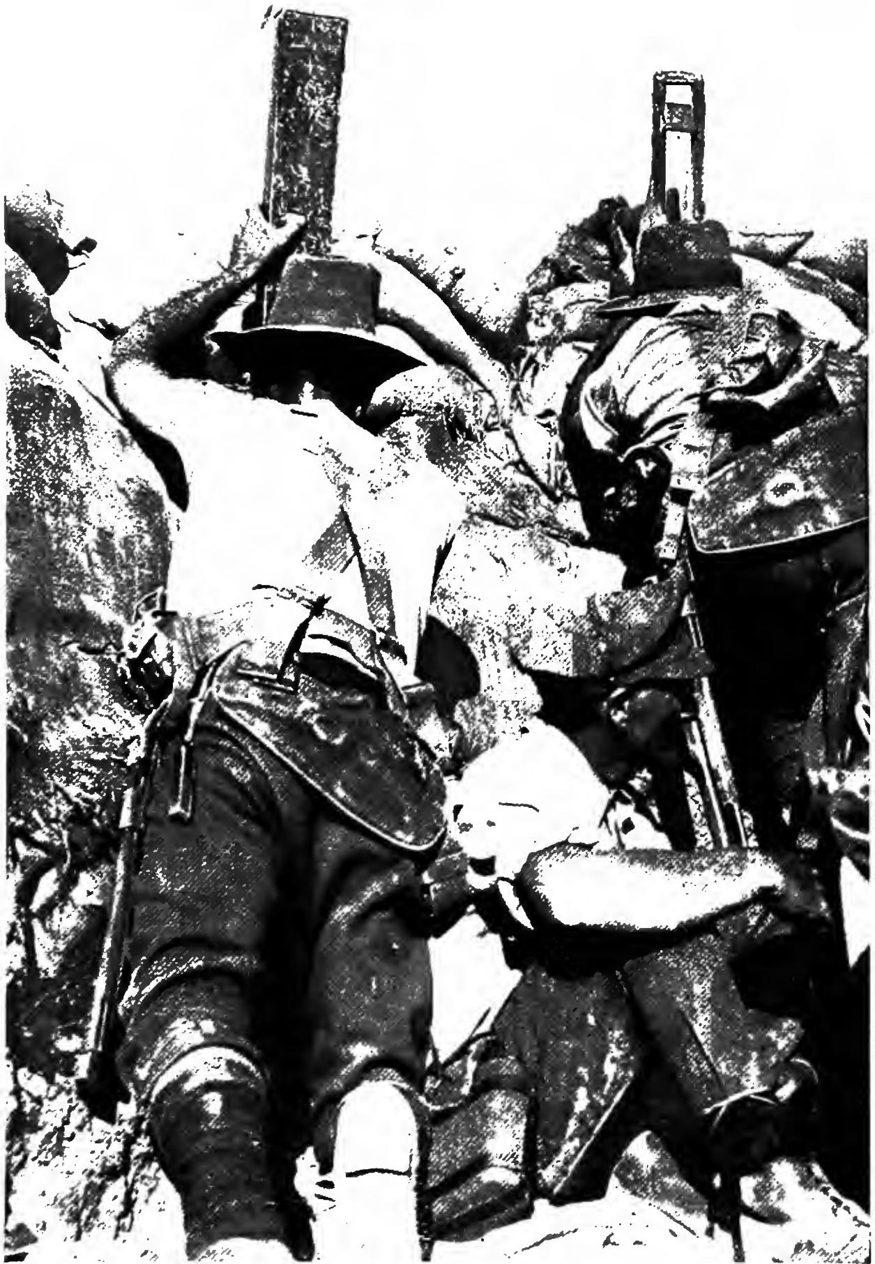
Inside an Australian trench, showing a man using a periscope rifle and another man keeping watch by means of a periscope
