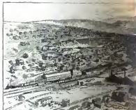
OIL CITY REPAIRS
