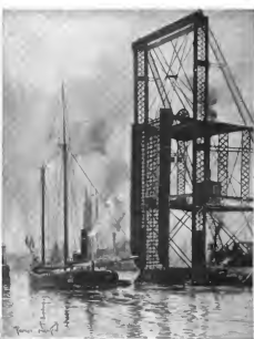
THE DRAWBRIDGE OVER THE HARLEM RIVER—THE LANDING OF THE CAR FROM HARLEM AT FORTRESS ROYAL.
