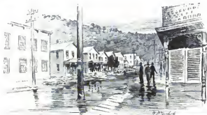
VIEW OF FLOOD ON SENeca STREET OIL CITY, ABOUT FIFTEEN MILES FROM BEFORE THE FIRE.
