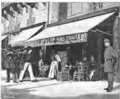
THE WINDOW IN WHICH BATAZOG WAS ARRESTED. Subsequently blown up.
