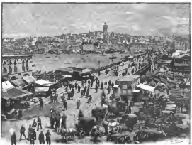
BRIDGE BETWEEN CONSTANTINOPLE AND STAMBOUL
