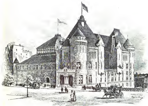
THE ARMORY FOR THE SEVENTY-FIRST REGIMENT N. G. S. N. Y.—J. H. THOMAS ARCHITECT.—DRAWN BY BLOOMER HANKEY.—[SEE PAGE 196.]
