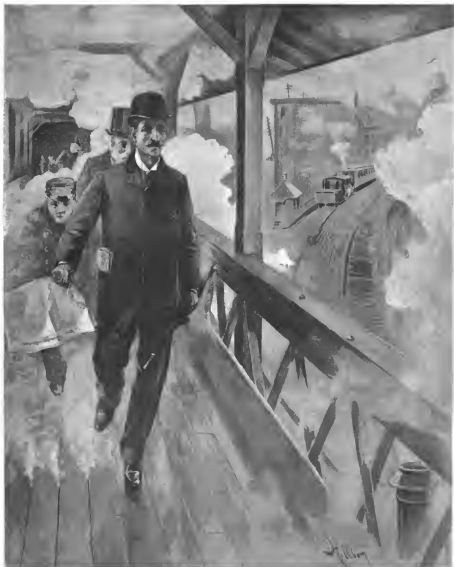
THE ELEVATED RAILROAD BRIDGE AT CHATHAM SQUARE.—Drawn by HENRY BILLING.—[See Page 223.]
