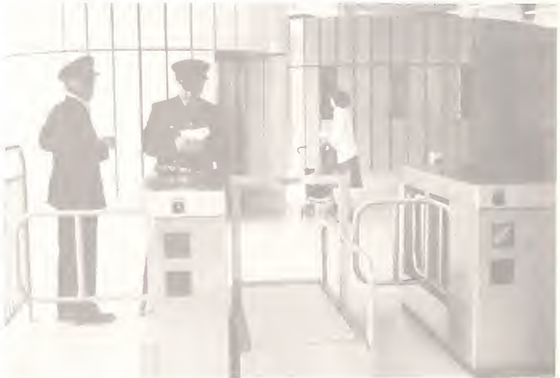
UMTA is assessing innovative foreign automatic fare collection equipment such as this passenger gate in Newcastle, England, to determine the potential for application on U.S. systems.
