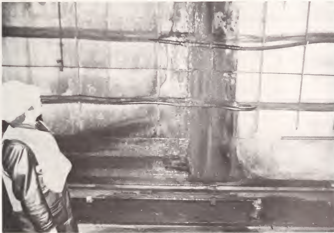
A WMATA study of water intrusion in tunnels addresses a problem common to most rail transit systems.
