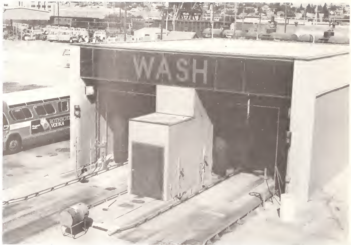
One recently completed NCTRP study dealt with transit bus washing equipment and procedures.
