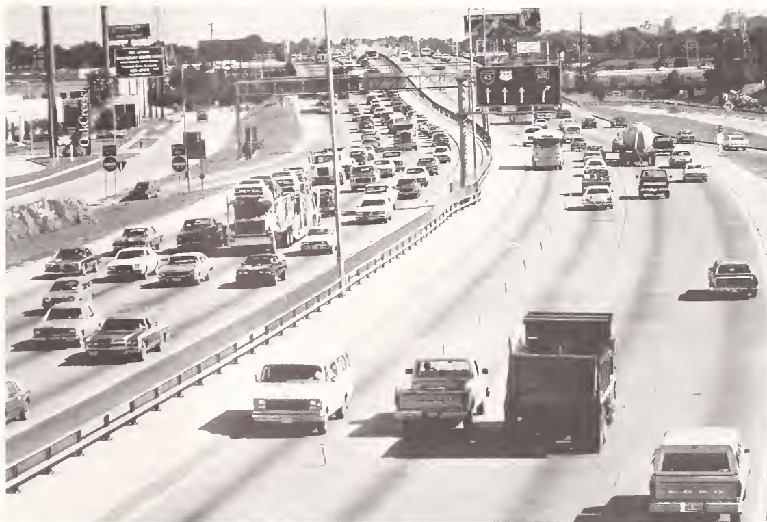
In Houston, Texas, the contra-flow bus and vanpool lane has significantly reduced travel times for these high-occupancy vehicles and has led to substantial increases in ride-sharing and transit use in the I-45 corridor (Host City Program participant).
