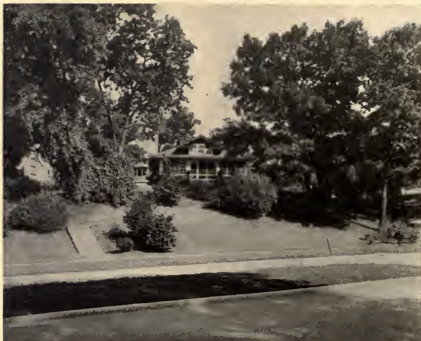
Fig. 15—A small home well located. Notice the arrangement of the front walk and how much better it is than a long flight of steps to the front door would be
