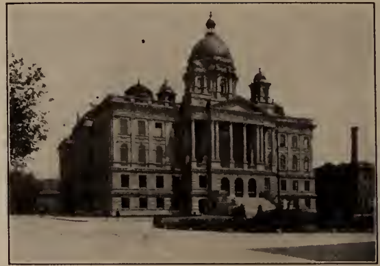
ONONDAGA COUNTY COURT HOUSE
