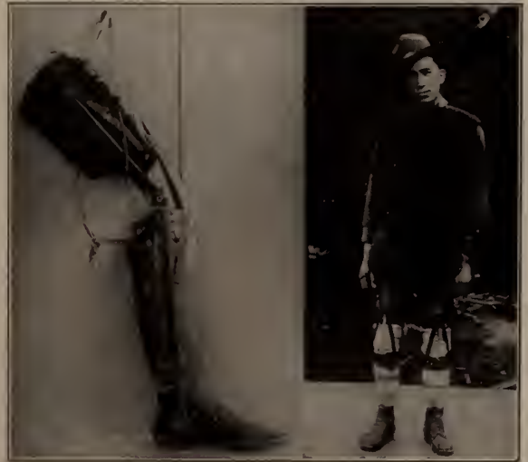
Plaster socket with paraffin liner. Constructed entirely in the hospital appliance shop.
