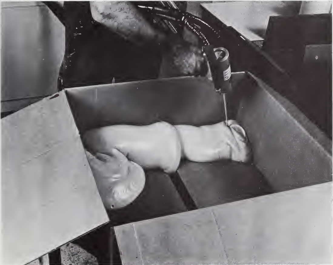
"Foaming in place."
