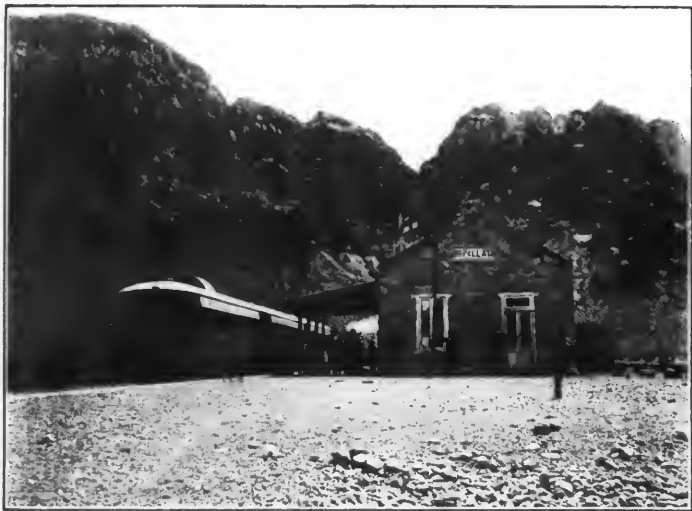
USPALLATA STATION, ARGENTINA, ON THE LINE OF THE TRANSANDINE RAILWAY.
