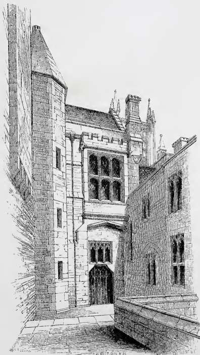
View of part of the Vicars' Hall from the Close, restored 1864.
