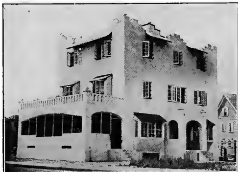
CEMENT HOUSE SOMEWHAT OF THE MEXICAN TYPE.
