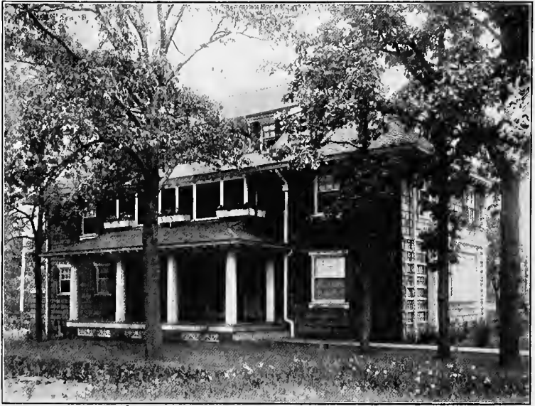
GALVANIZED IRON GUTTER AND CORNICE.
