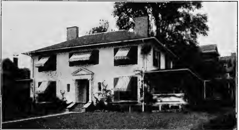
SHINGLE ROOF WITH HANGING METAL GUTTER.
