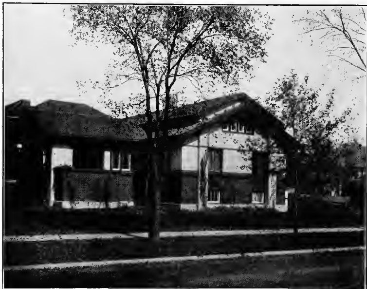
GREEN STAIN ON SHINGLES AND ROUGH-SAWED TRIM.
