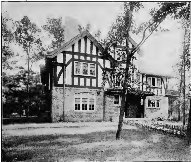
ENGLISH "TIMBER-WORK" HOUSE AS BUILT IN AMERICA.
