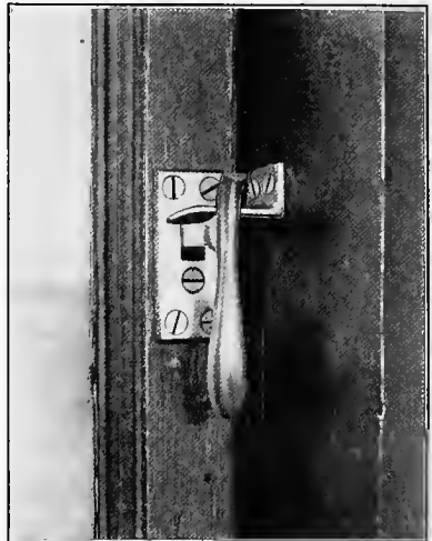
EXCELLENT PATTERN OF CASEMENT WINDOW FASTENER.
