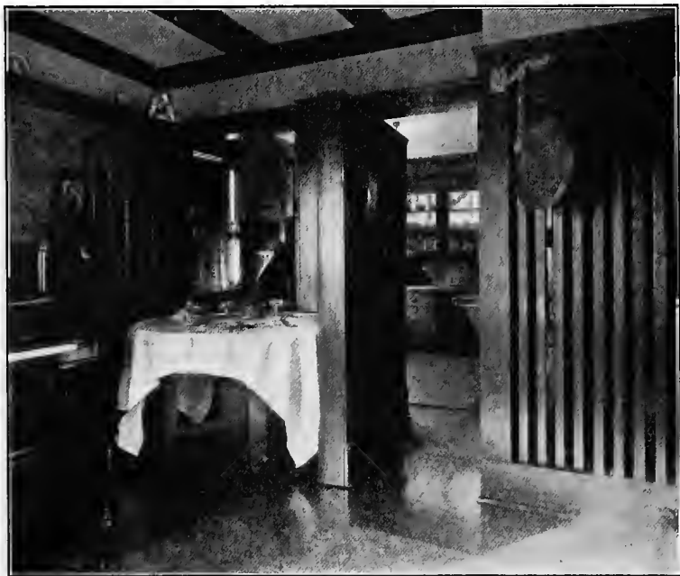
SWINGING PARTITION BETWEEN LIVING ROOM AND KITCHEN. (See floor plan on preceding page.)
