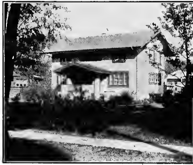
CEMENT-PLASTERED HOUSE OF MODERATE COST.
