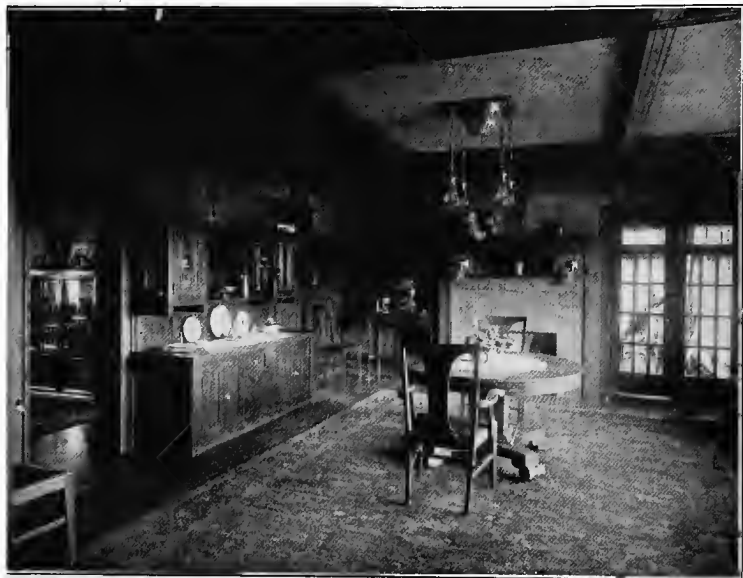
DINING ROOM OPENING ON AN INCLOSED PORCH.
