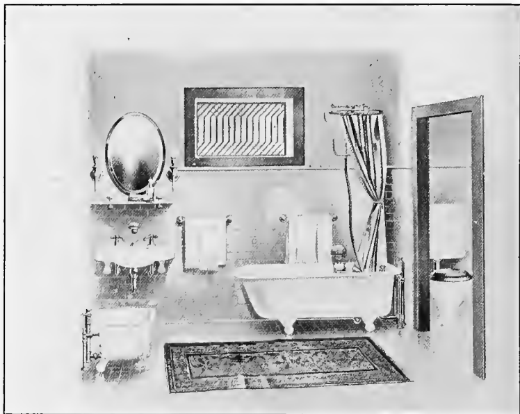
A WELL ARRANGED BATH ROOM; WATER CLOSET IN A SEPARATE COMPARTMENT.
