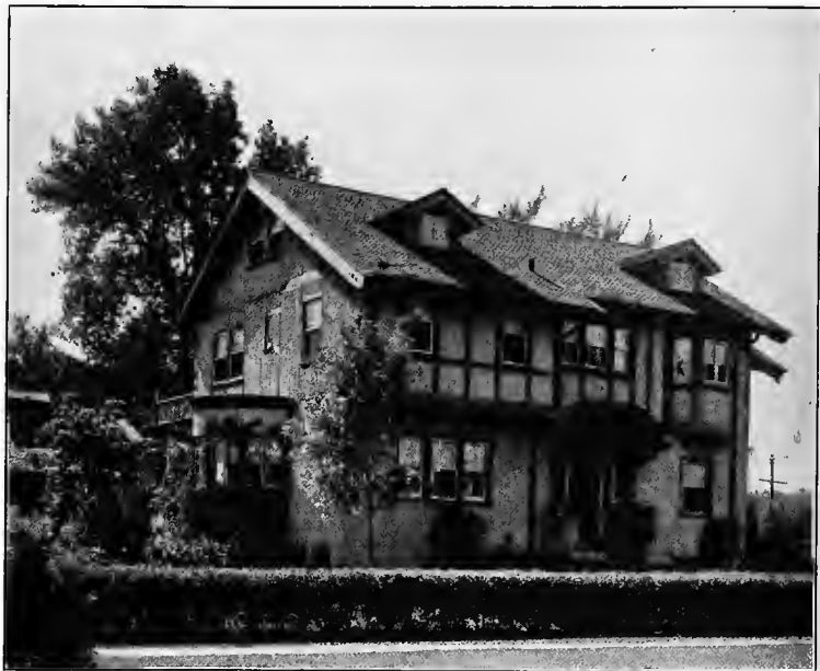
BUILT-IN GUTTERS LINED WITH COPPER.
