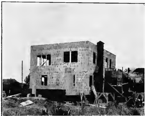
TILE HOUSE IN PROCESS OF CONSTRUCTION.
