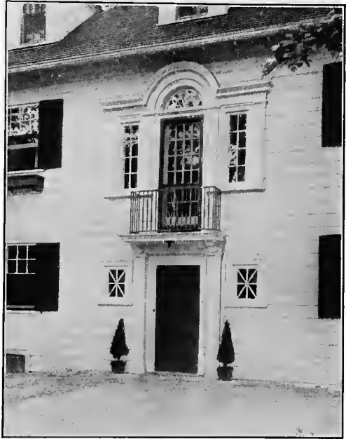
BALCONY OVER A MAIN ENTRANCE.
