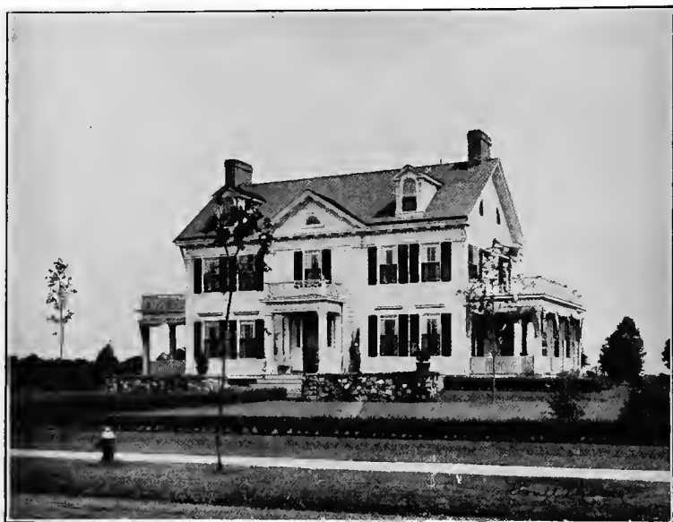
MODERN ADAPTATION OF OLD COLONIAL HOUSE. Lionel Moses, II, Architect.
