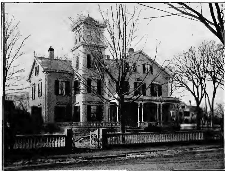
OLD HOUSE BEFORE REMODELING.
