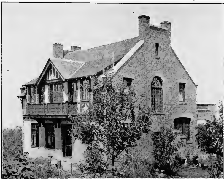
PLUMBING STACKS EXTENDING ABOVE ROOF.
