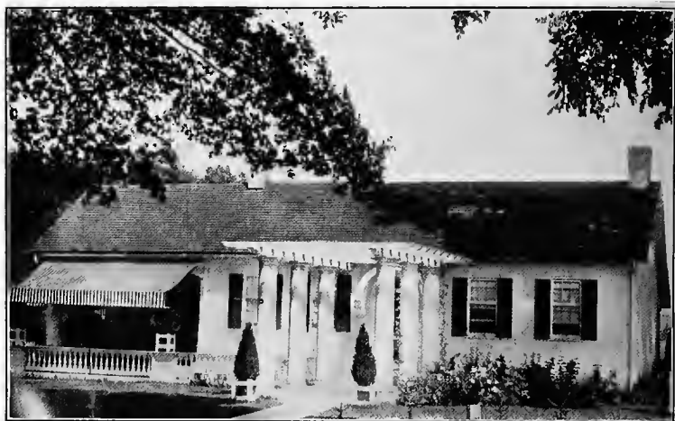
LITTLE BRICK HOUSE WITH NEW PORCH AND PERGOLA.
