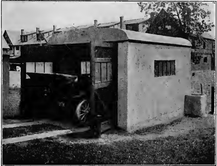
METAL FRAME PLASTERED GARAGE.
