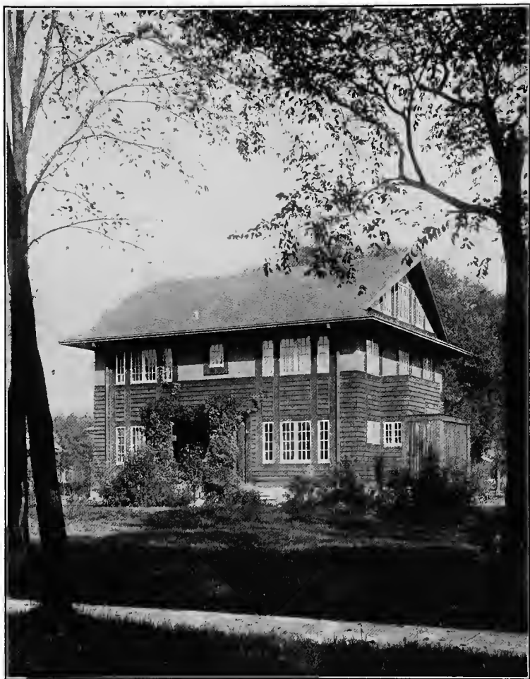
THE CHARM OF ROUGH BROWN SIDING AND GRAY PLASTER. Tallmadge and Watson, Architects.
