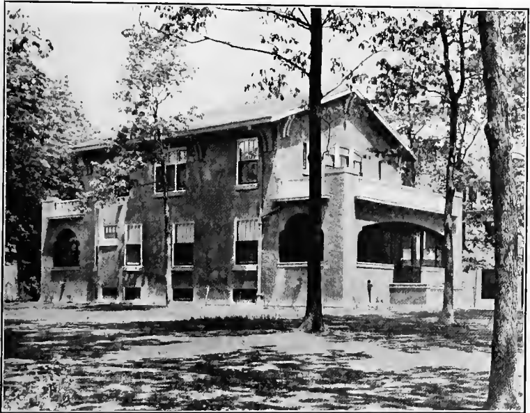
STEEL FRAME HOUSE COMPLETED.
