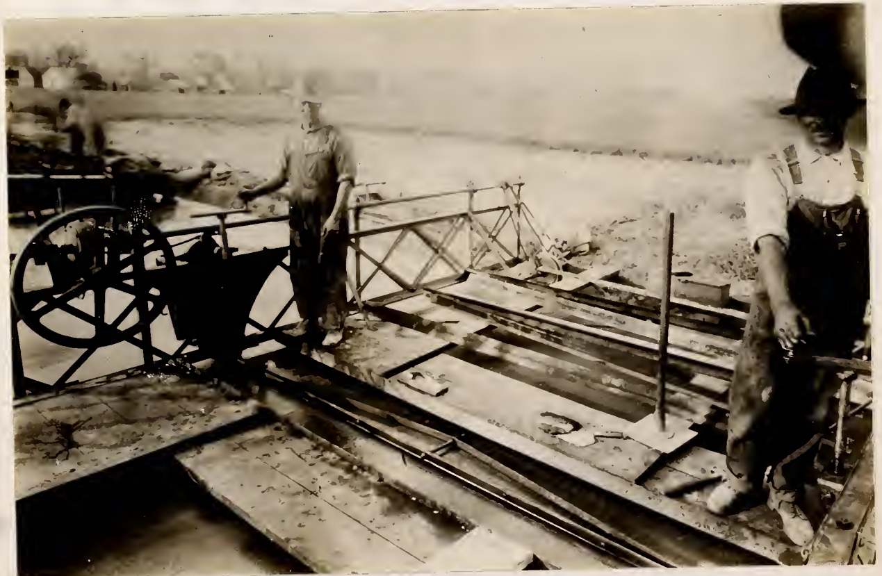
FIG. IV - SHOWING 10-FOOT SECTION OF MOLD BEING FORCED INTO THE CONCRETE.
