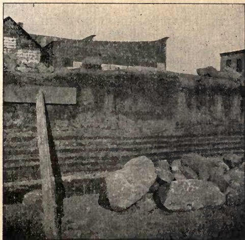
FIG. 47. Stratified Clay, Sediments of Bottom of Lake Agassiz. Excavation in City of Mayville. Photograph by the Author.
