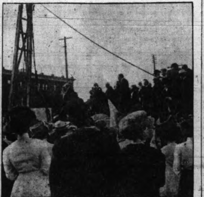
CORNER STONE OF Y. M. C. A. BEING LAID. The new home of the local association is being erected at the corner of Viv and Blanchard streets, and will be a five-storey building, 114 feet by 100 feet.
