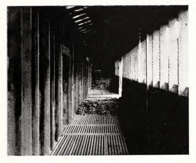
Above cut shows our drying room for drying corn on the ear. Underneath the slat bottom floor is ten 1½ inch steam pipes which artificially drys the corn. This insures high germination and the seed will always keep without heating.
