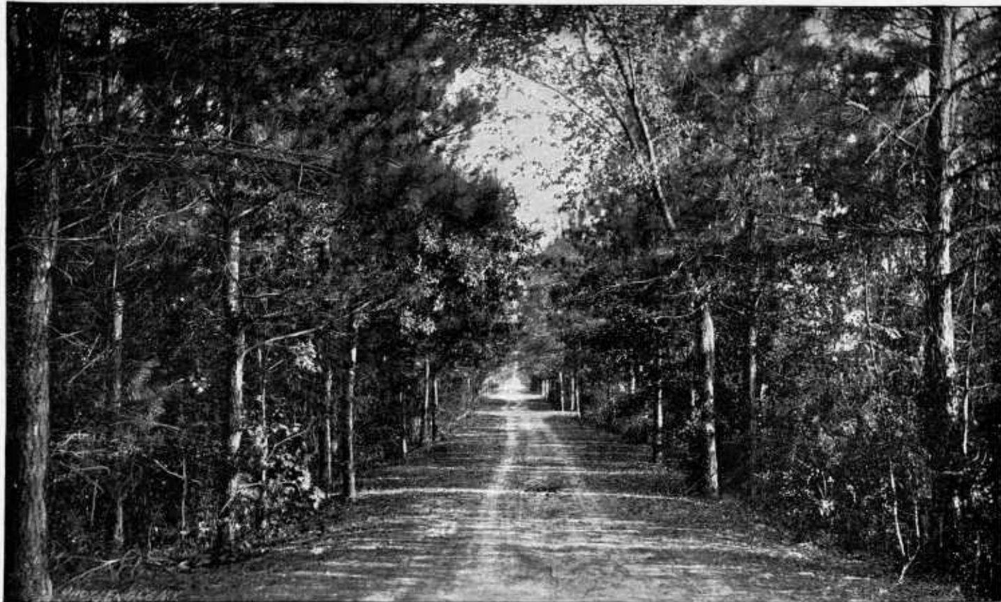
SECTION OF SHELL ROAD 8 MILES LONG, WILMINGTON TO WRIGHTSVILLE, NEW HANOVER COUNTY, N. C.
