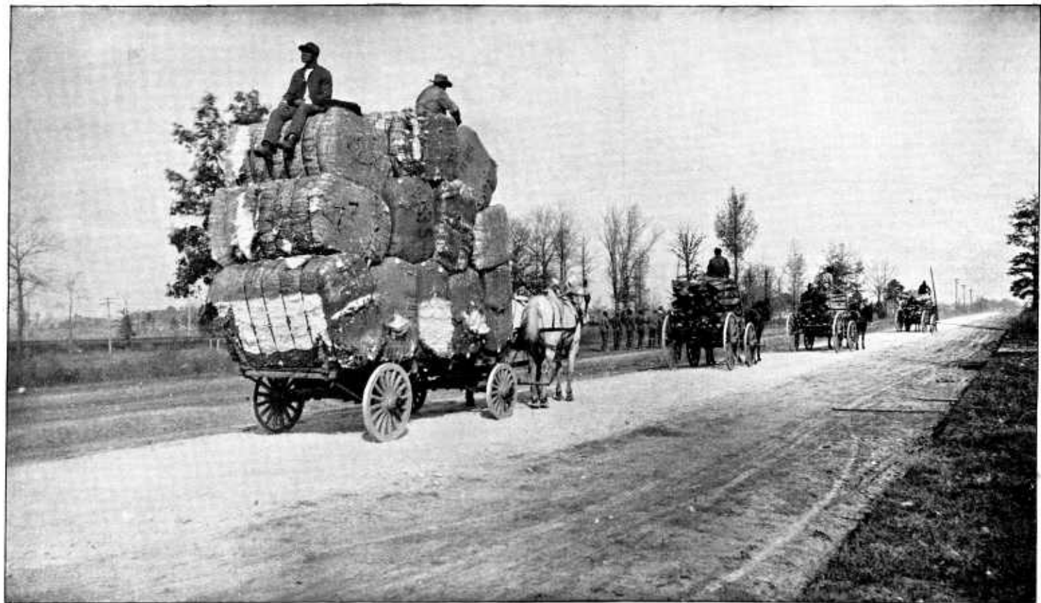
SECTION OF MACADAMIZED ROAD NEAR CAMDEN, N. C., SHOWING SIZE OF LOADS HAULED OVER IT.
