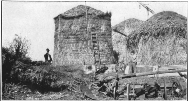
FIG. 2.—"TROJES" CONSTRUCTED OF CORNSTALKS. Sometimes stalks and husks are used for covering.
