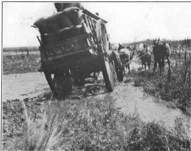
FIG. 1.—HAULING GRAIN TO RAILROAD STATION. The roads at times are impassable.
