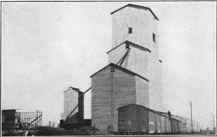
FIG. 2.—COUNTRY GRAIN ELEVATOR RECENTLY CONSTRUCTED IN ARGENTINA.
