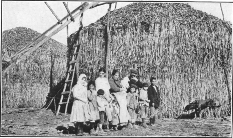
FIG. 1.—COMPLETED "TROJES," CONSTRUCTED OF CANE STALKS. Italian farmer and family are seen in the foreground.
