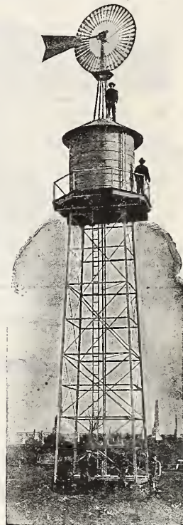
Substructure and Tank with Windmill.
