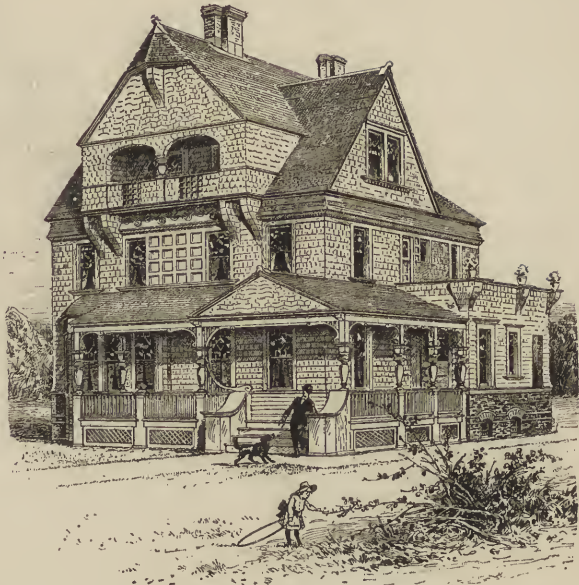
A Builder's Design.—Example of crude work.
