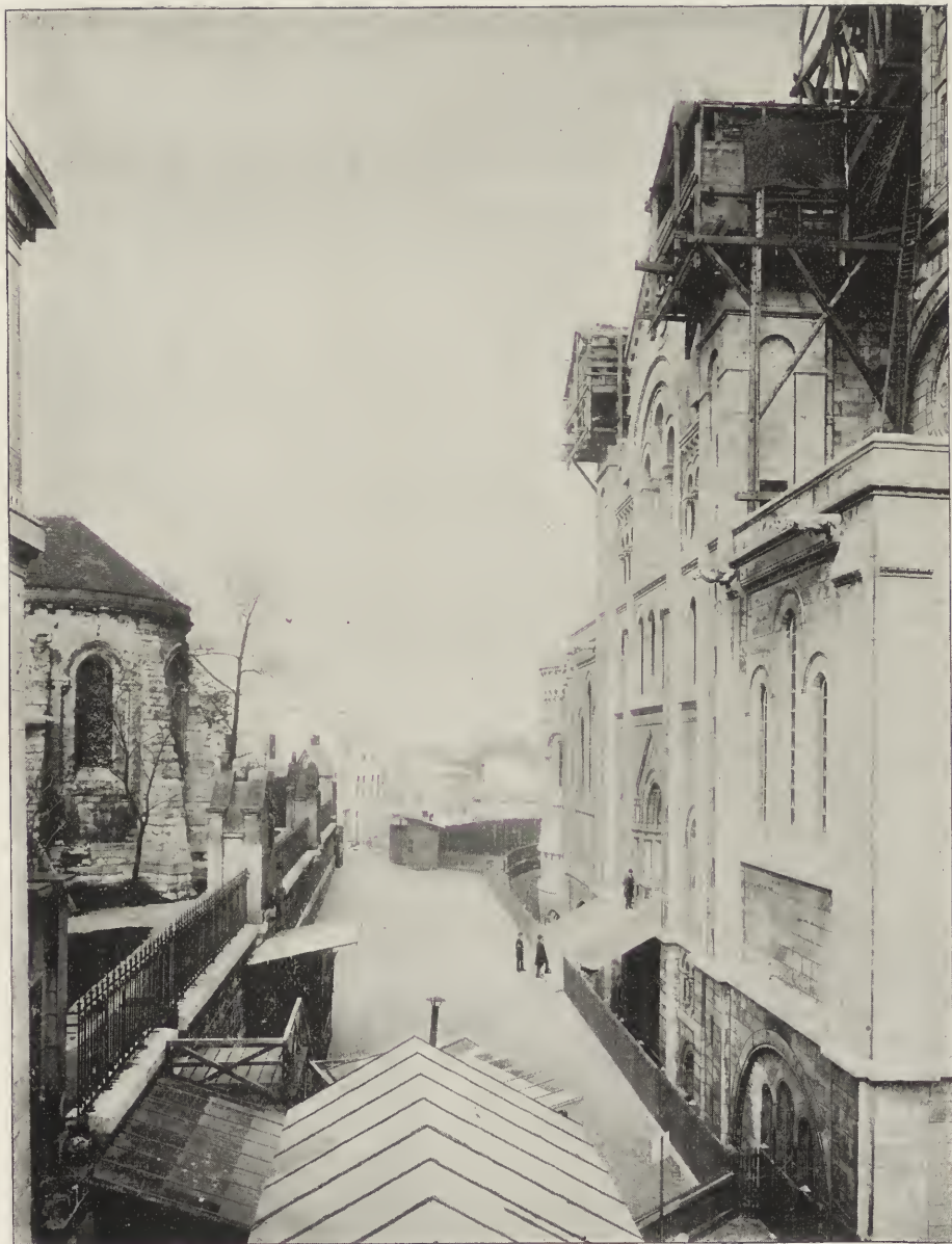
VIEW OF WEST FAÇADE.
