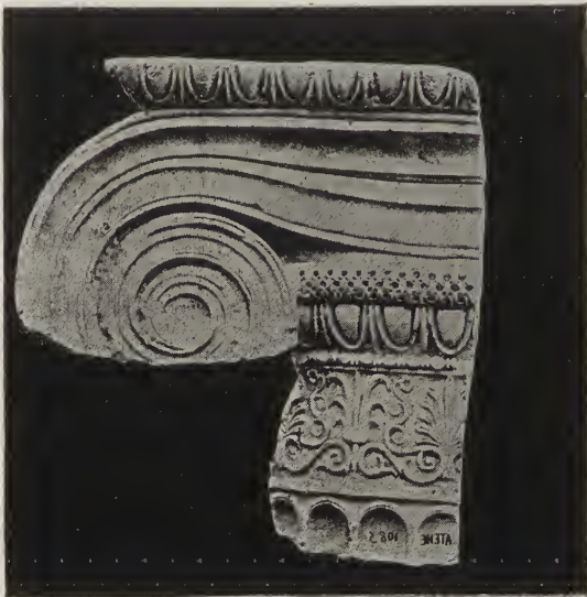
Cast of a portion of an Ionic capital ; from the Erechtheum. Necking ornament of anthemions, two lines of the egg-and-dart moulding, multiple form of the guilloche.
