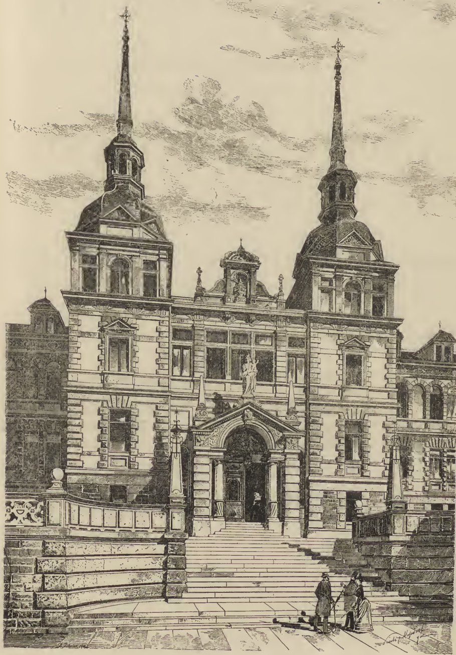
MIDDLE BUILDING OF ST. MARY'S HOSPITAL.
