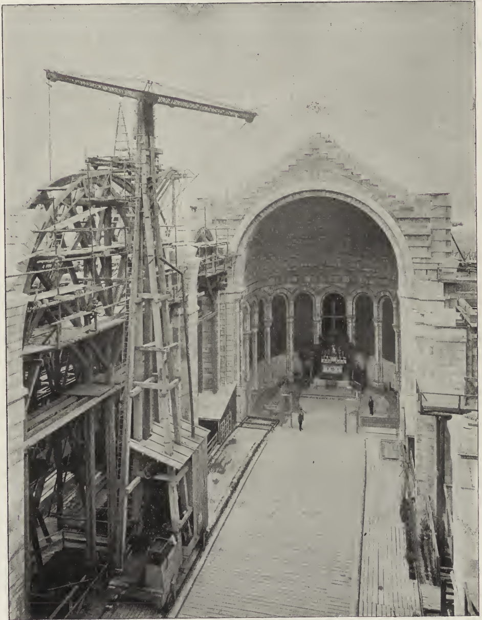
VIEW ALONG THE NAVE.
