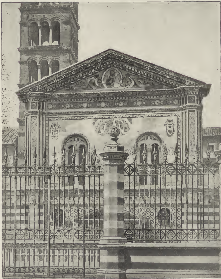
CHURCH OF STA. PUDENTIANA, ROME. Showing facade in mosaic.
