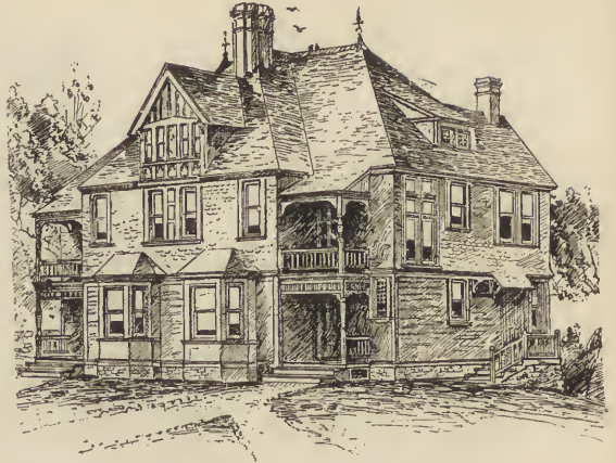
A Builder's Design.—Example of crude work.
