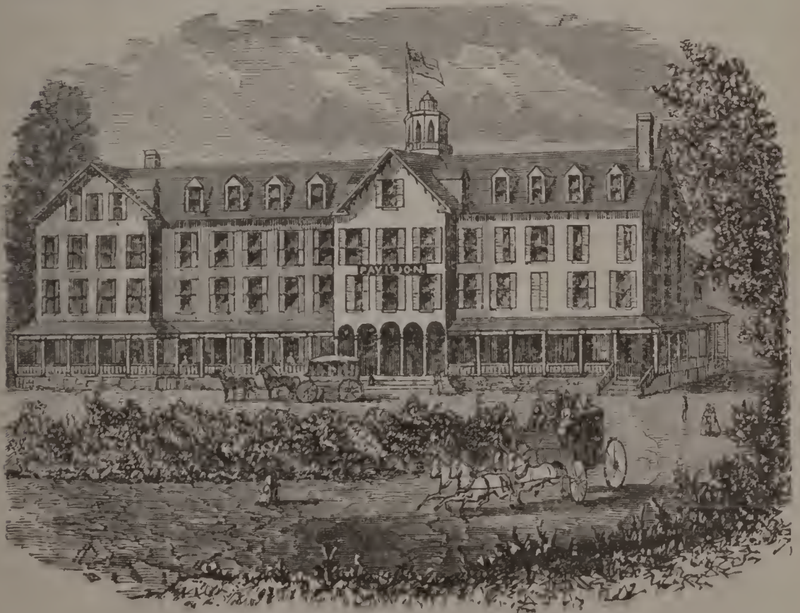
THE WOLFEBOROUGH PAVILION,
