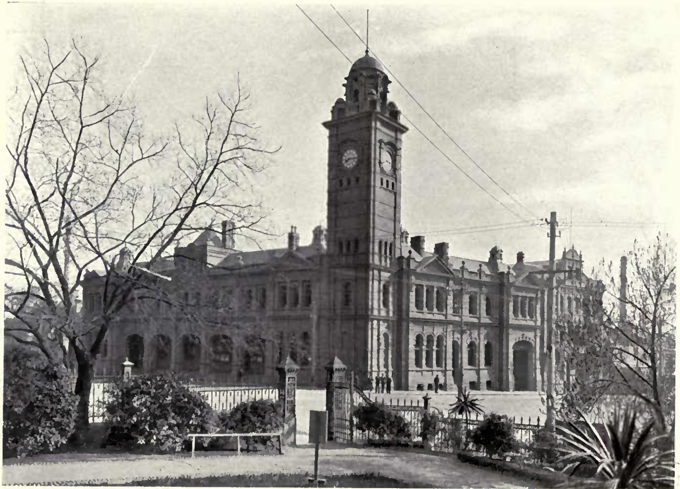
BASE COURSES, RISDON QUARRIES. UPPER STRUCTURE, BRYN ESTYN QUARRIES. (G.P.O., HOBART, TAS.)
