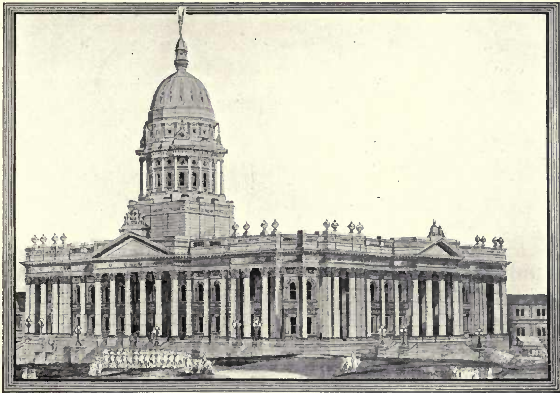
BASE COURSES AND STEPS, WEST ISLAND GRANITE. UPPER STRUCTURE, KAPUNDA GREY MARBLE. (PARLIAMENT HOUSE, ADELAIDE, S.A.)
