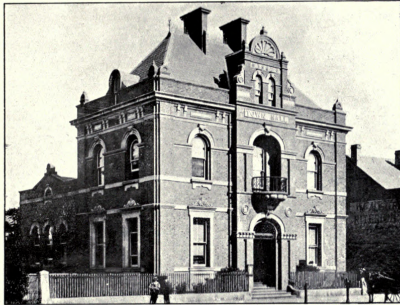
BUNDANOON SANDSTONE DRESSINGS. (GOULBURN TOWN HALL, N.S.W.)
