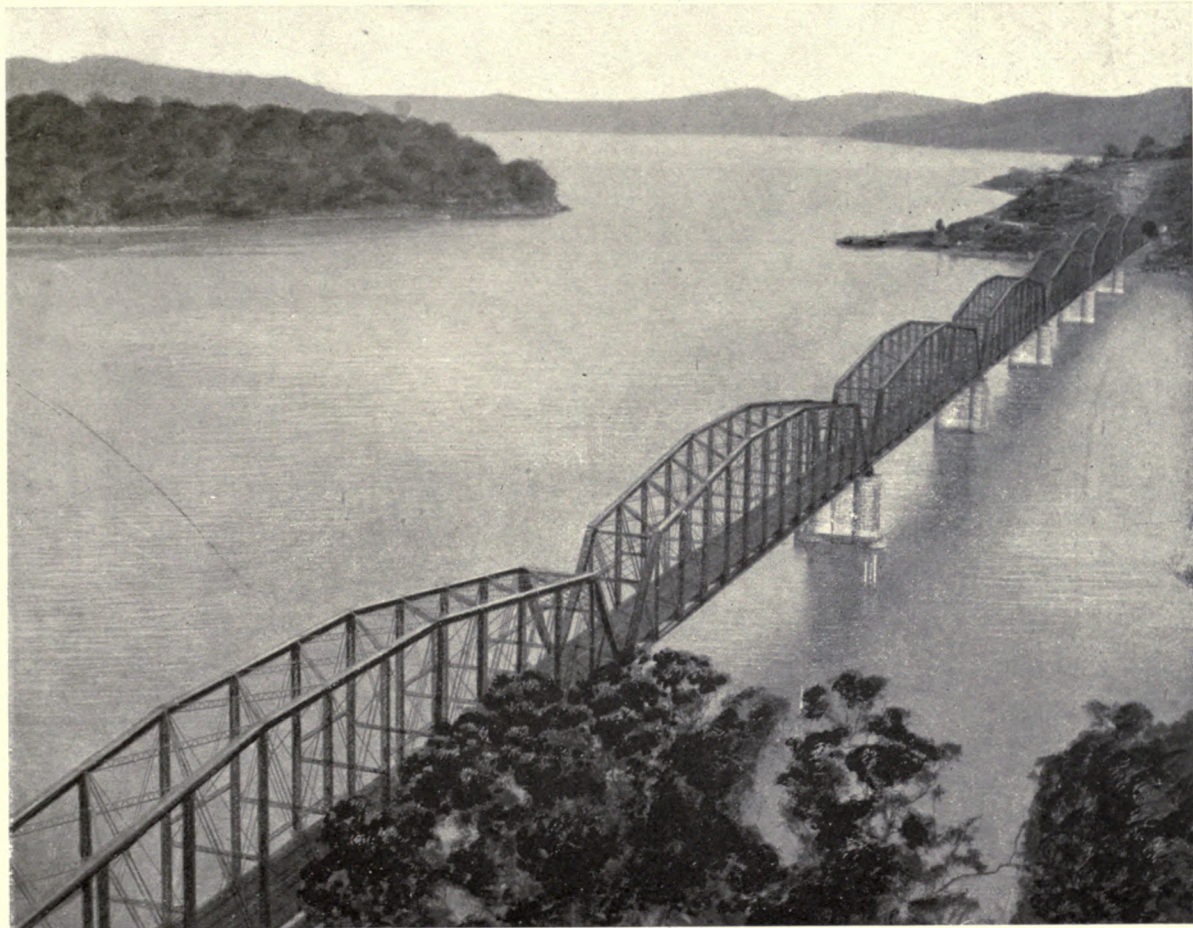
PIERS OF BOWRAL TRACHYTE. (HAWKESBURY RIVER BRIDGE, N.S.W.)
