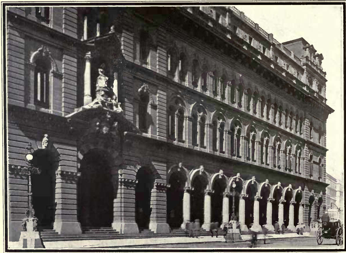
COLUMNS OF MORUYA AND MONTAQUE ISLAND GRANITE. (COLONNADE, GENERAL POST OFFICE, SYDNEY, N.S.W.)
