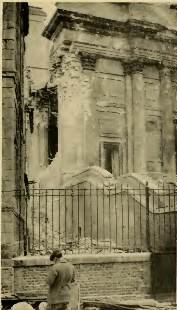
Effects of shell fire and explosive bombs over the great portals of Arras Cathedral
