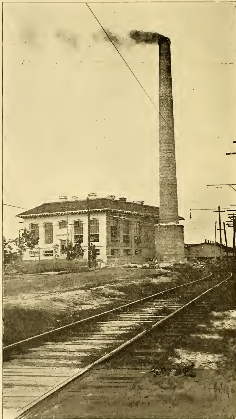
POWER HOUSE OF GULFPORT & MISSISSIPPI COAST TRACTION COMPANY.
