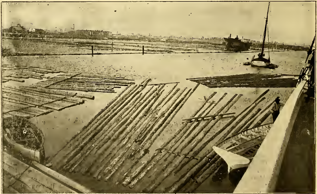
PILING IN THE BASIN AT GULFPORT AWAITING SHIPMENT TO PANAMA.
