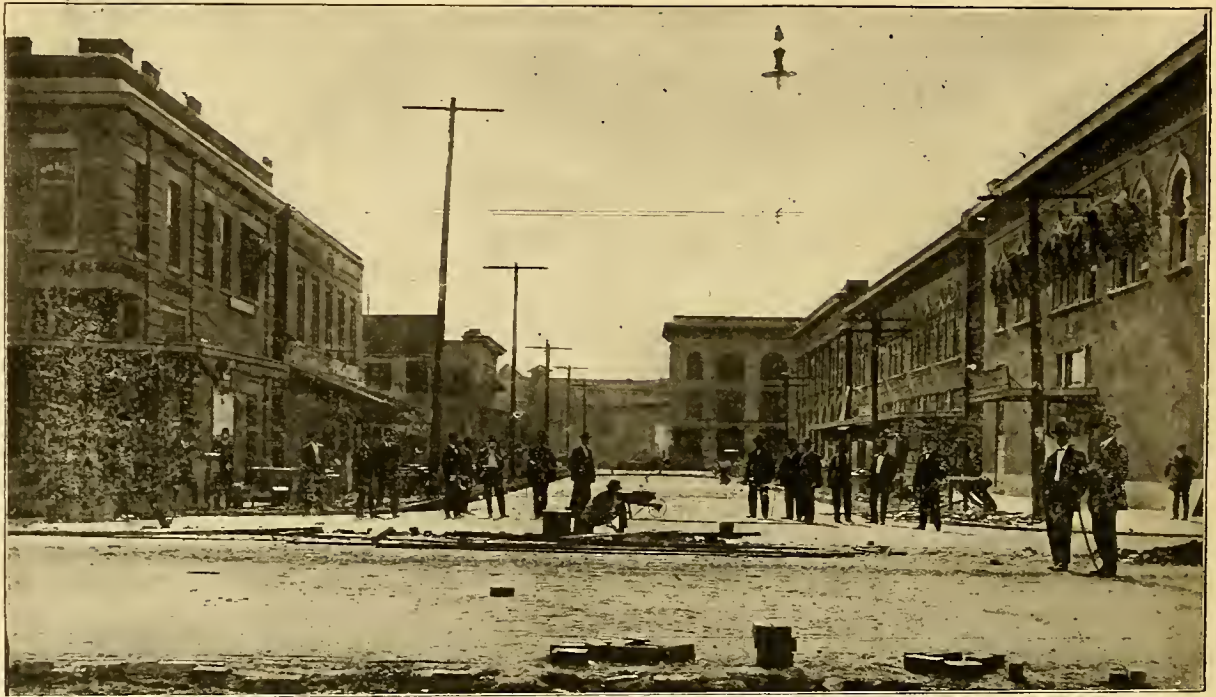
PAVING WITH VITRIFIED BRICK AT THE INTERSECTION OF 26TH AVENUE AND 14TH STREET.
