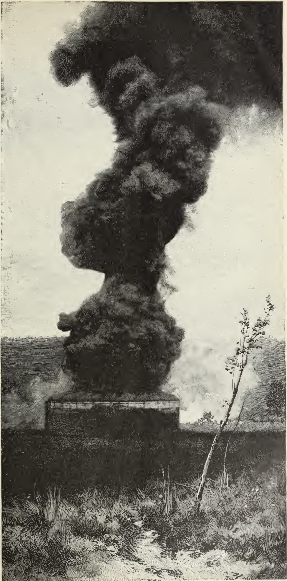
A BURNING TANK.
