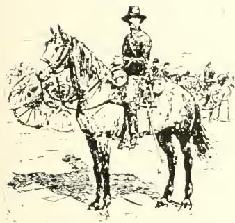
Battery on Drill.
