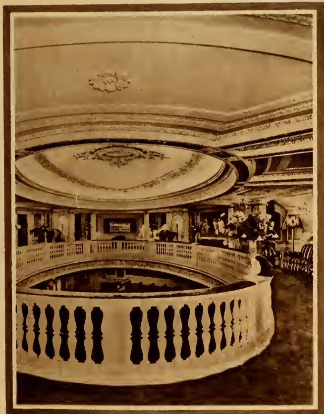
GENERAL VIEW OF THE MEZZANINE, THE RIVOLI
