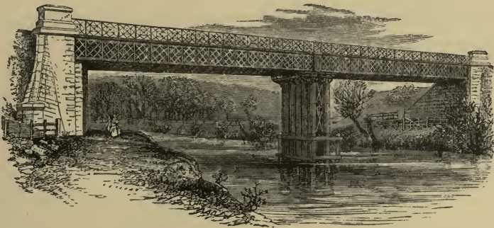
BRIDGE OVER THE AVON, NEAR BATH.
