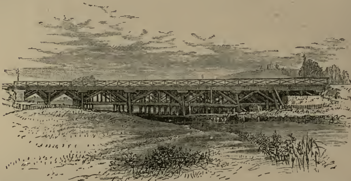
THE VIADUCT AS IT WAS (MIDLAND RAILWAY). NIPHANY, NEAR SKIPTON.
