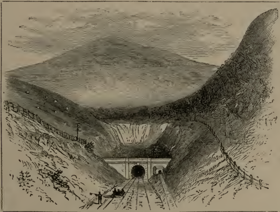
DOVE HOLES CUTTING CLEARED.
