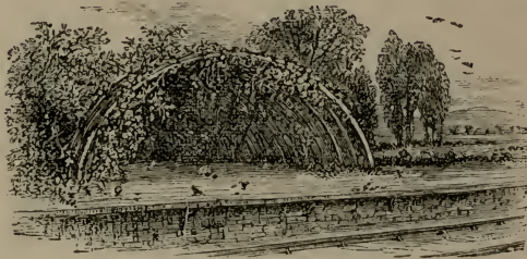
A WELSH RAILWAY STATION.
