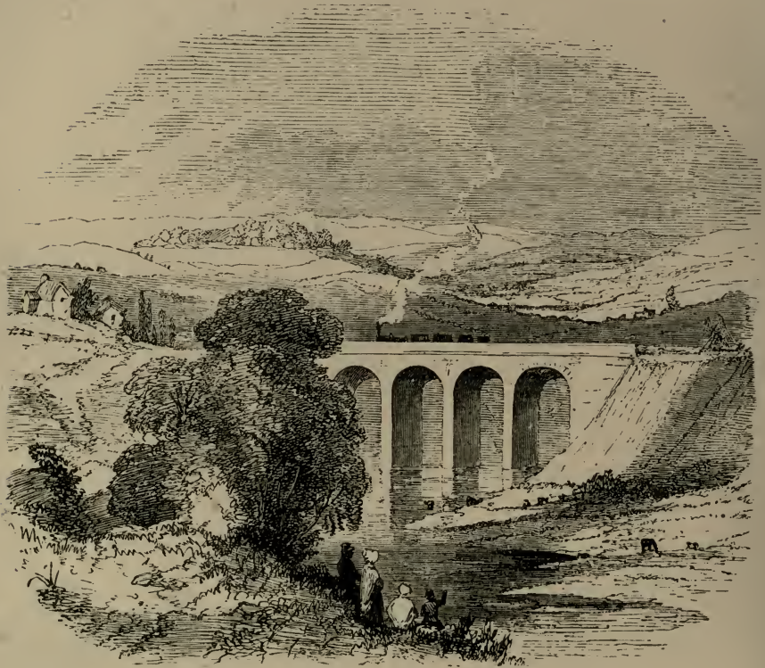
DRYFE SANDS VIADUCT.
