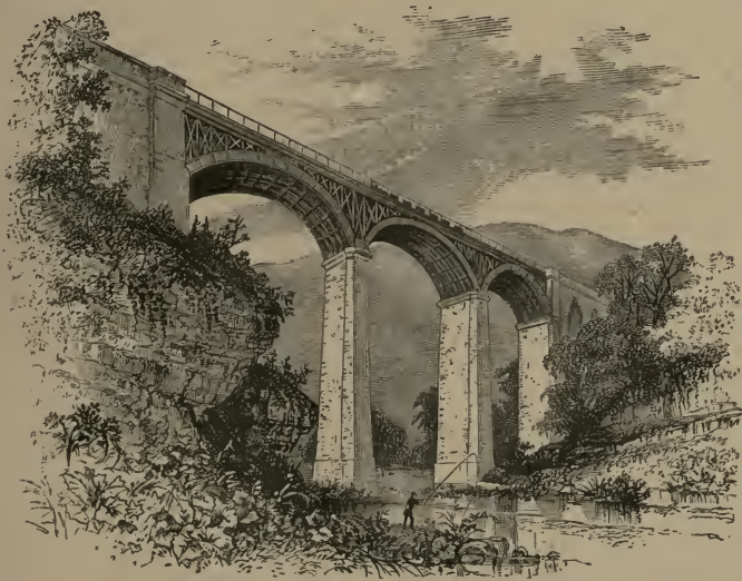
MILLER'S DALE VIADUCT.
