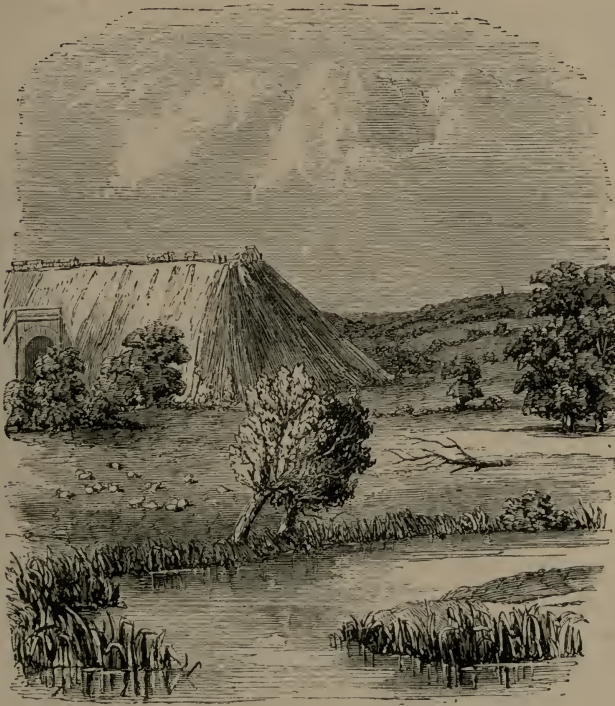
MAKING THE WOLVERTON EMBANKMENT.
