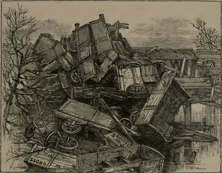
ACCIDENT TO AN EMPTY COAL TRAIN.
