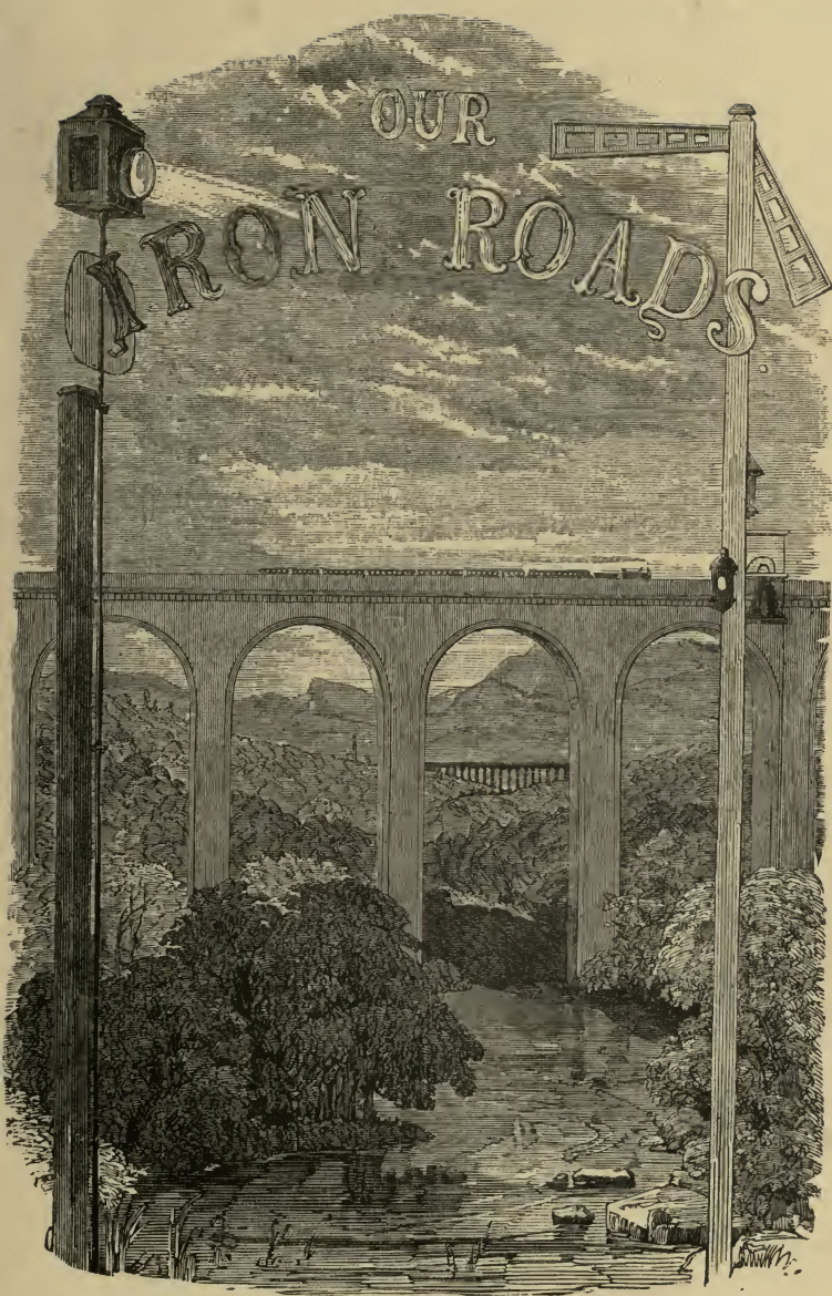
VALE OF LLANGOLLEN VIADUCT.
