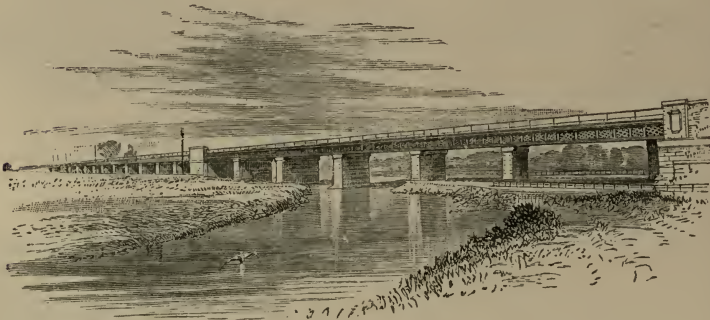
THE VIADUCT AS IT IS (MIDLAND RAILWAY). NIPHANY, NEAR SKIPTON.
