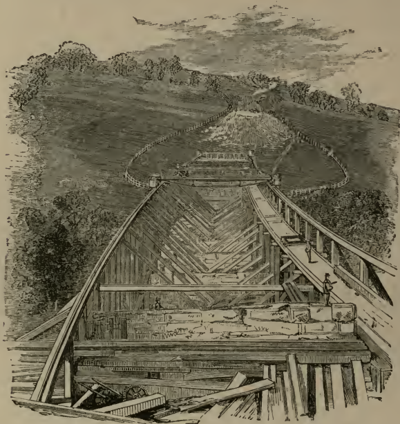
SMARDALE VIADUCT IN COURSE OF CONSTRUCTION.
