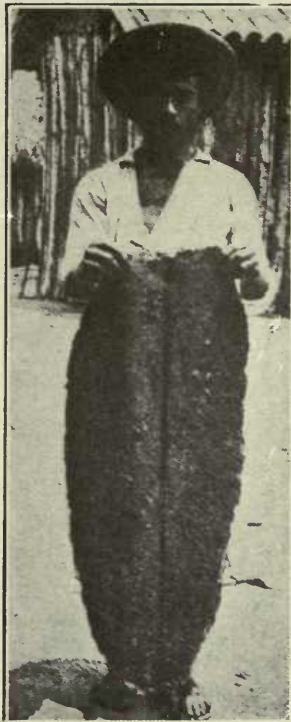
FIG. 19—PREPARING RUBBER ON OJA BLANCA LEAVES REMOVING RUBBER SHEET
