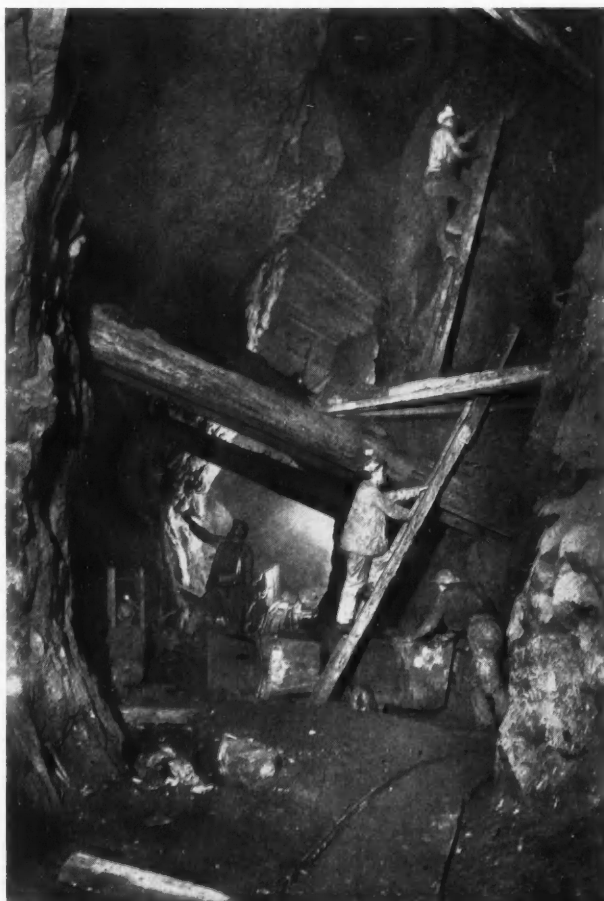
2. THE 180 AT EAST POOL MINE.
